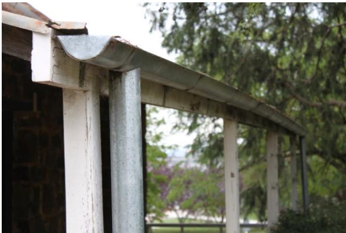
Figure 3.10 Half round gutter at front verandah. (Source: GML 2013)
