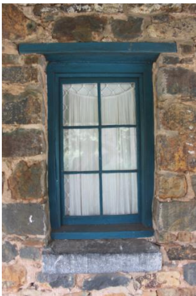
Figure 3.11. Front verandah window with timber lintel, hardwood frame, six-pane sash and shaped stone sill. (Source: GML: 2013)
