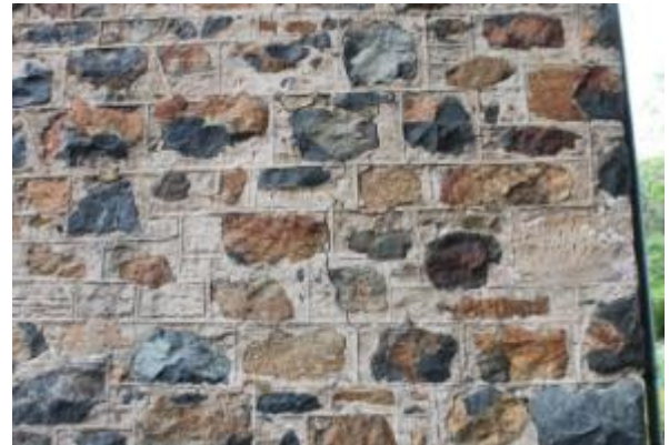
Figure 3.14 Raised pointing and structural crack in 1888 wall. (Source: GML 2013)
