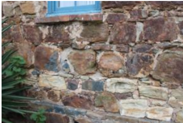
Figure 3.13 Deeply eroded mortar in 1859 west wall. (Source: GML 2013)
