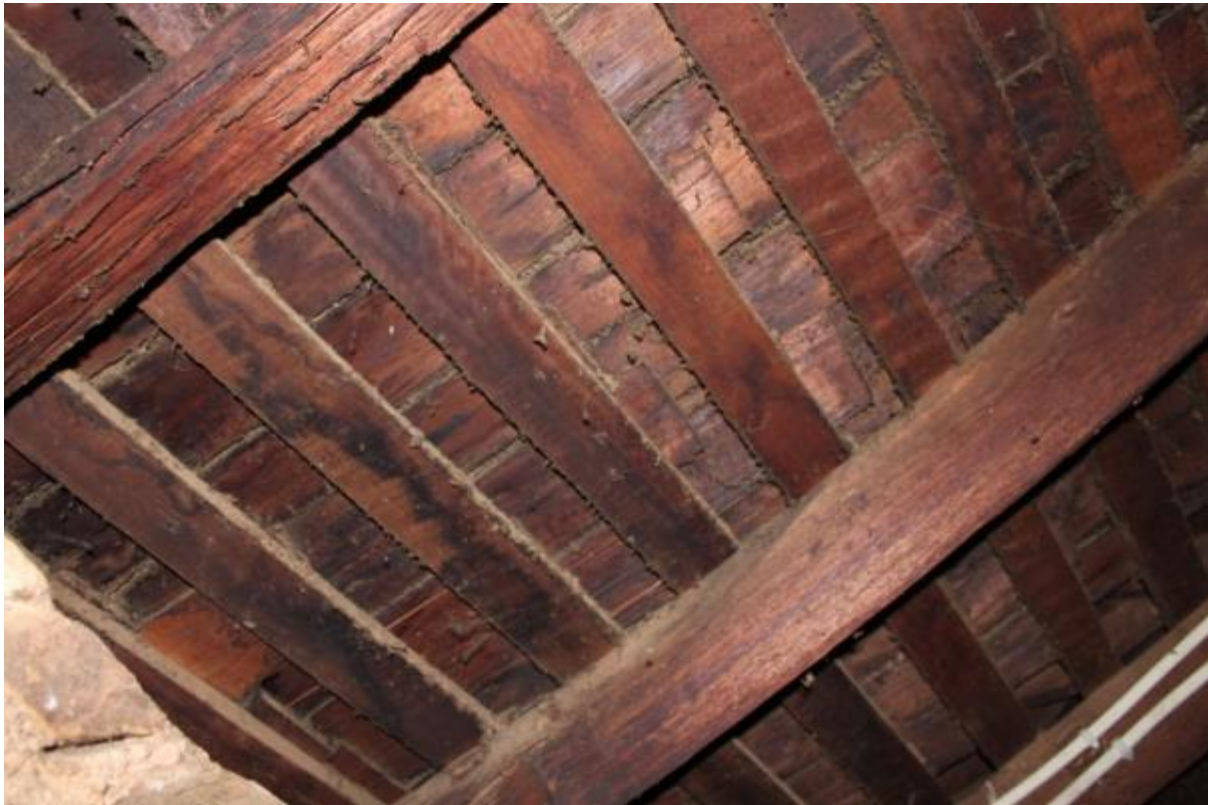
Figure 3.7 Underside of roof above parlour showing 1859 split rafters, sawn battens and shingles. (Source: GML 2013)
