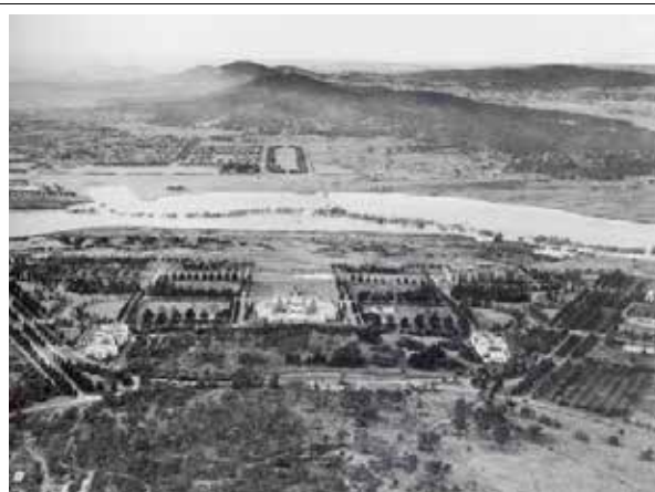
Figure 3.26 1956 view looking north towards Mount Ainslie showing Lake Burley Griffin under construction. The newly constructed Administrative Building (now the John Gorton Building) is shown to the right of Old Parliament House near the lake. (Source: National Capital Authority)
