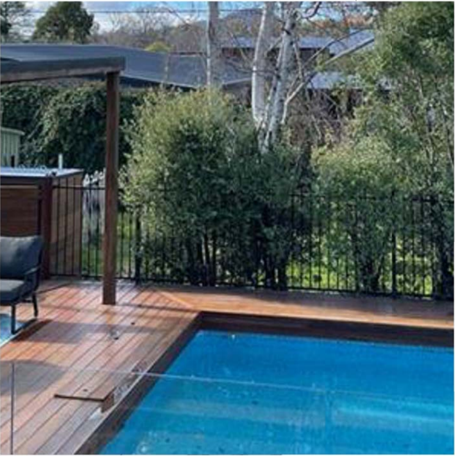
TD - TIMBER DECK TIMBER DECK USED FOR POOL DECKING RECYCLED FROM EXISTING SPOTTED GUM POOL DECKING.
