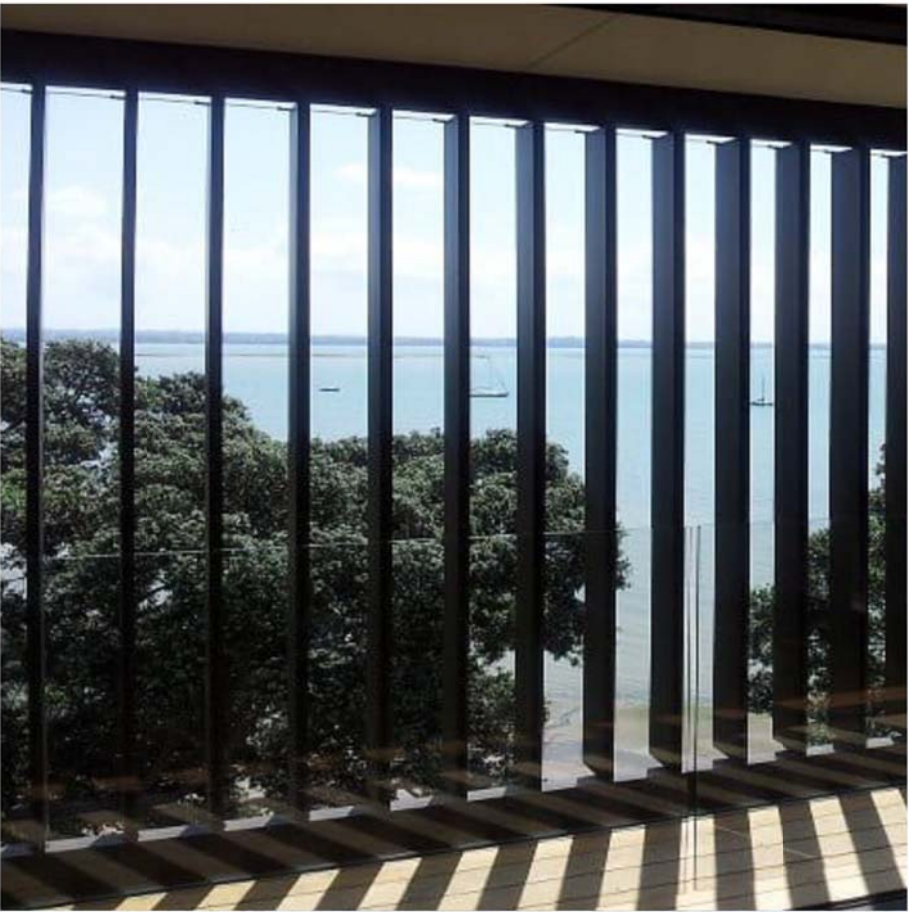
OL - OPERABLE LOUVER ALUMINIUM CHARCOAL FINISH. USED FOR PRIVACY AND SOLAR SCREENING TO LIVING
