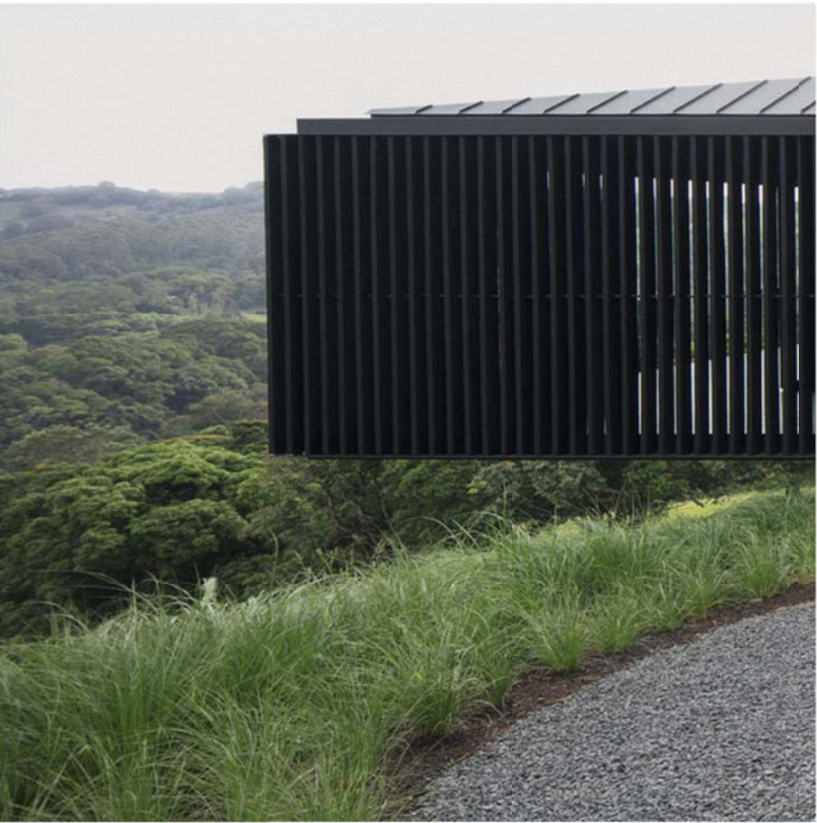
LO - LOUVER BLADES NATURAL DARK TIMBER FINISH. USED FOR SCREENING TO NATIONAL CIRCUIT
