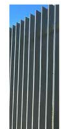
FEN 1 FENCE TYPE 1 3200 HIGH PALISADE CONSTRUCTION POWDERCOATED TO MATCH ADJACENT WALL COLOUR
