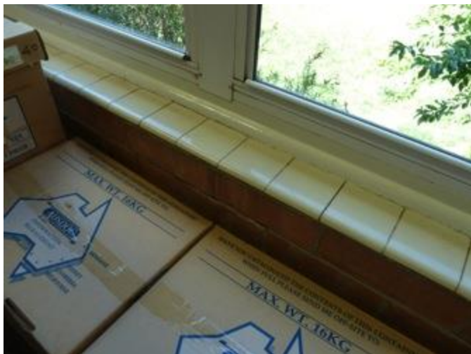
Figure 17. Glazed sill tiles and face brickwork in the former northeast verandah of the former TB Ward – Building 1 in 2013
