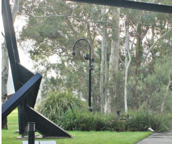
Figure 3.53 Pole lighting with integrated CCTV on a swan neck in the Sculpture Garden. (Source: Phillips Marler, 2017)
