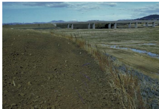
Figure 2.8 Detail of the Aspen Island constructed platform showing the rock foundation and topsoil, c1960–1962. (Source: National Library of Australia, PIC P2214/211)
