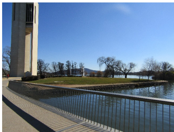
Figure 3.2 View from the footbridge towards the northern portion of the island. One of the three grassed mounds are visible. (Source: GML, July–August 2019)
