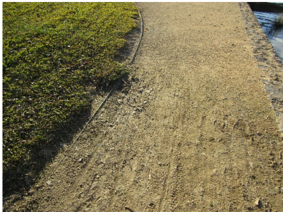
Figure 3.18 Detail of gravel path with metal edging strip evident on the left, and the rubble-wall island edge on the right. (Source: GML, July–August 2019)
