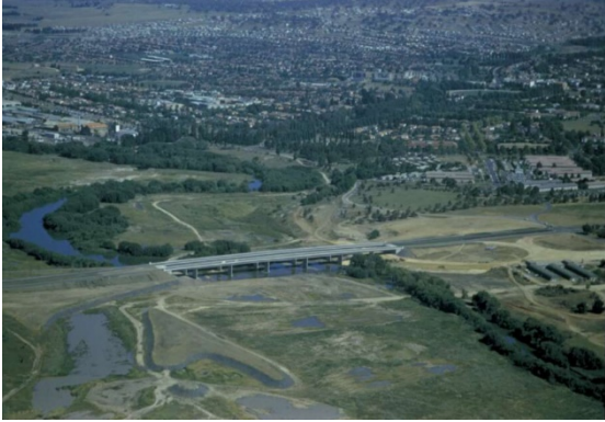
Figure 2.9 Aerial, c1962 of the completed Aspen Island platform prior to the filling of the lake. (Source: National Library of Australia, PIC P2214/162)
