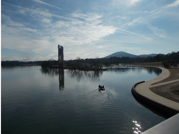
Figure 3.46 View north from Kings Avenue Bridge. (Source: GML, July–August 2019)
