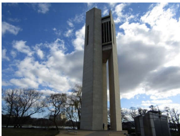
Figure 3.22 View westward toward Carillon. (Source: GML, July–August 2019)
