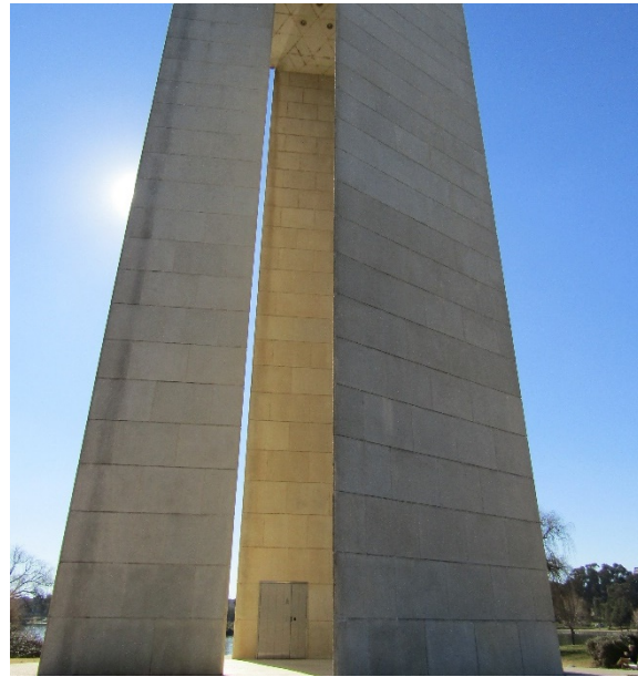
Figure 3.27 View east towards the base of the Carillon. (Source: GML, July–August 2019)
