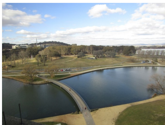
Figure 3.15 View of the footbridge from the Carillon, which shows its curved shape. (Source: GML, July–August 2019)
