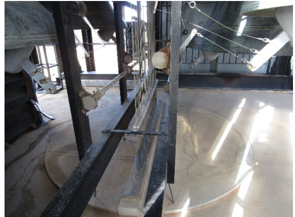
Figure 3.33 View within the Bell Chamber showing the wires and linkages that connect with the clavier on the level below. (Source: GML, July–August 2019)
