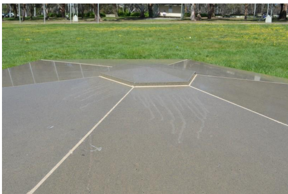
Figure 3.20 Detail of the capping stone. The white runoff visible on the cap is from the application of a new sealant.
