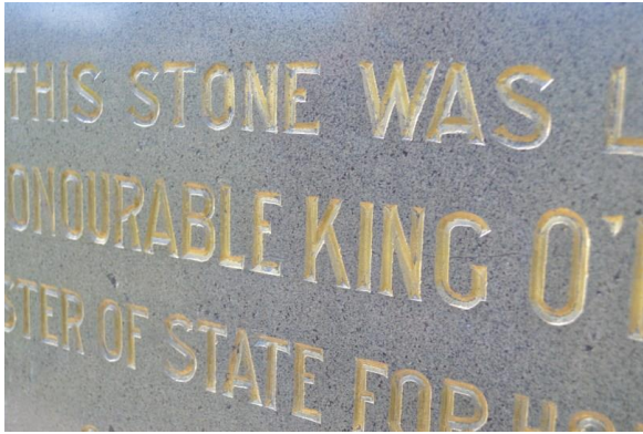
Figure 3.16 Detail of the incised lettering on the foundation stones. The use of both gold leaf and metallic pigment paint has caused a dull and mottled appearance to the letters.
