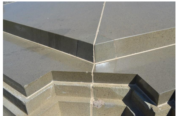
Figure 3.19 Detail of the horizontal and sloped capping. The difference in colour and shine between the base and capping is evident.
