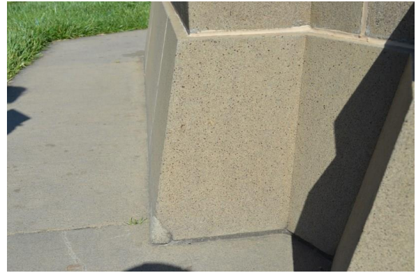
Figure 3.17 Detail of the paving and angled skirting stone showing patching work to the chipped base.
