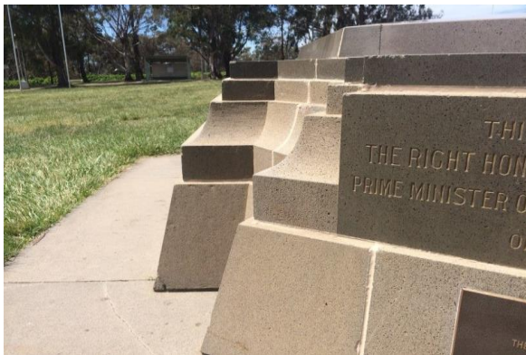
Figure 3.18 Detail of the decorative moulding on top of the angled skirting. The decorative moulding is between the foundation stones.
