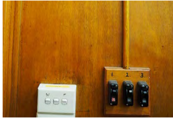
Photograph 3.37 Timber switchboard fixed to original in-built cupboards
