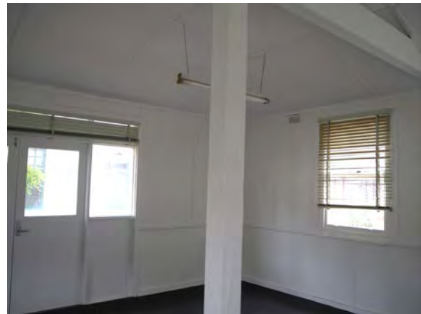
Photograph 3.79 Inside the south-east portion of Store 17, timber beam and simple strut system
