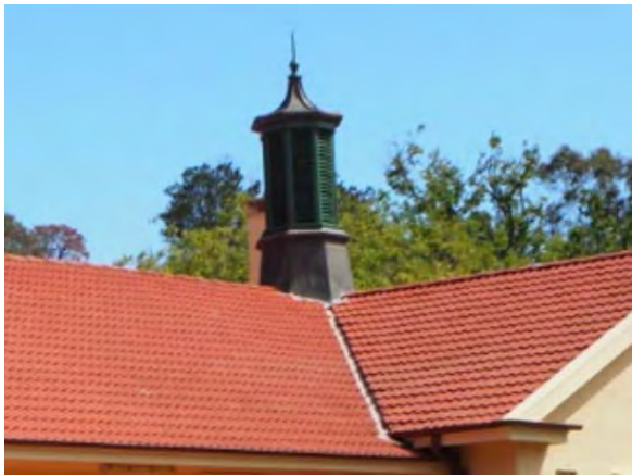
Photograph 3.95 Bronze and timber turret at apex of gabled roof elevation
