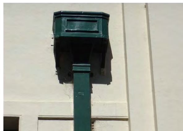
Photograph 3.63 Cast iron downpipe from the AFS building
