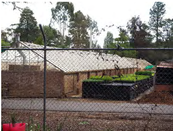
Photograph 3.140 Plant House at Yarralumla Nursery with brick wall supporting gabled roof
