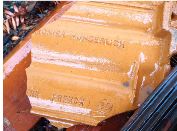
Photograph 3.57 Close-up of roof tile, 'Monier Wunderlich' French tiles
