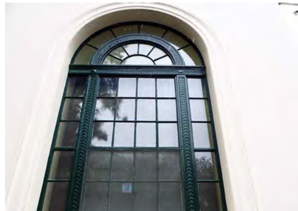
Photograph 3.24 Timber framed arched window
