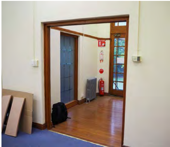
Photograph 3.67 Timber framed frosted picture window, originally door to Papers room
