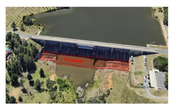
(g) The dam dissipator has five bays, adjacent to the five gates. Bays 1 and 5 are located 3m (10') higher than Bays 2 and 3. Bay 4 provides a sloping transition between the different slab elevations of Bay 3 and Bay 5 as shown in the following image.
