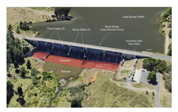
(b) The Dam is operated to maintain the level of the Lake within a narrow tolerance. The water levels are maintained at full supply level through use of two independent water release systems, the sluice gates and flood gates.
