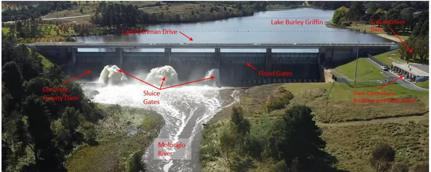
Figure 2.3 General arrangement of Dam
