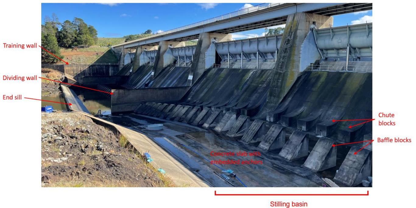
Figure 2.4 General layout of Scrivener Dam dissipator
