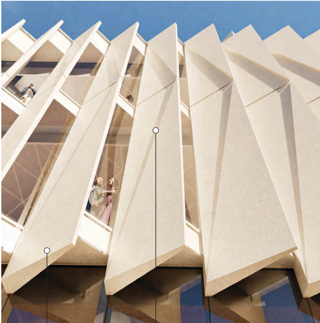
Serrated Folding Look in Façade Articulation to Create Dynamic Triangulated Shadows
