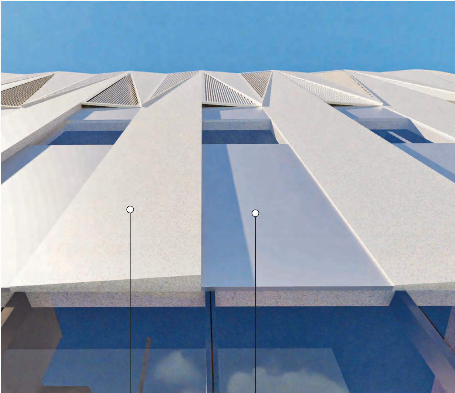
Shadowbox Detail, Low-E Glass with Back Panel Aluminium or Colorback Glass to match Interpon - White Stone
