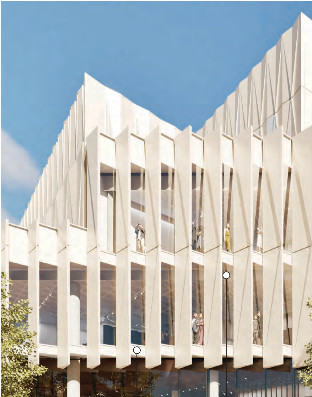
Shadowbox Detail, Low-E Glass with Back Panel Aluminium or Colorback Glass to match Interpon - White Stone
