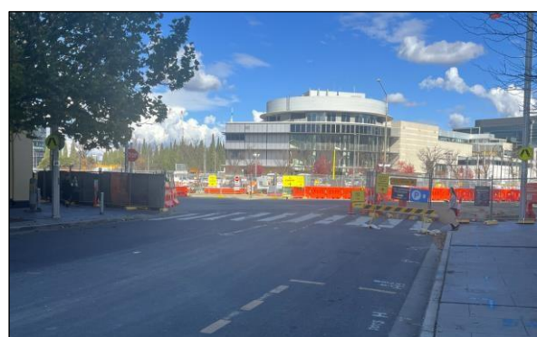
Photograph 4: The site as viewed from the north side of London Circuit looking west.
