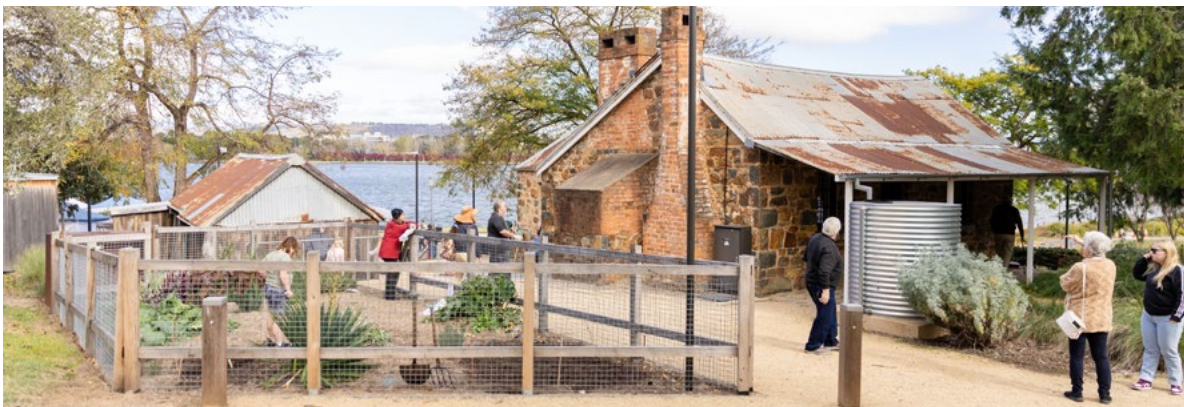
Blundells Cottage. Credit: National Capital Authority
