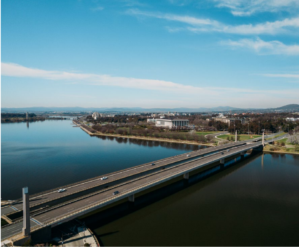
Commonwealth Avenue Bridge. Credit: Tim Bean
