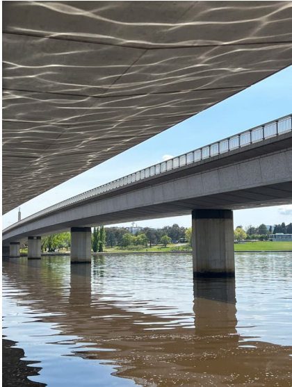
Figure 117: View of southbound bridge.
