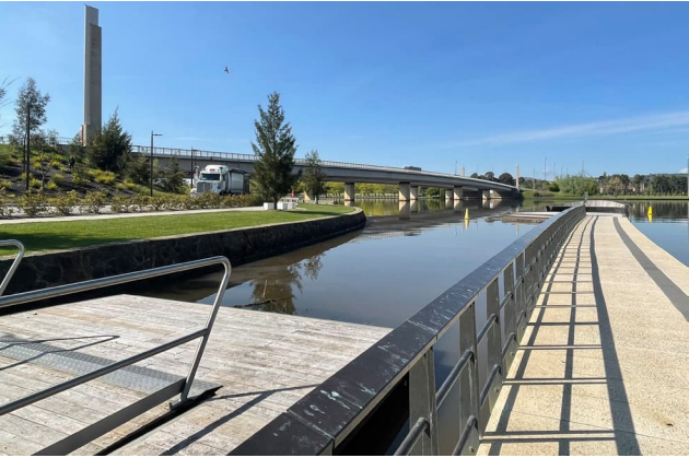
Figure 63: Commonwealth Avenue Bridge viewed from Henry Roland Park
