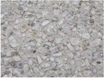
Figure 49: White precast concrete panel with exposed white Quartz aggregate.
