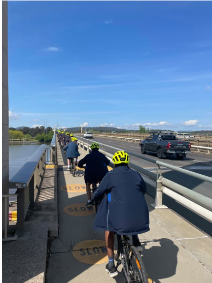
Figure 89: Pedestrian/ cycleway pinch point southbound.
