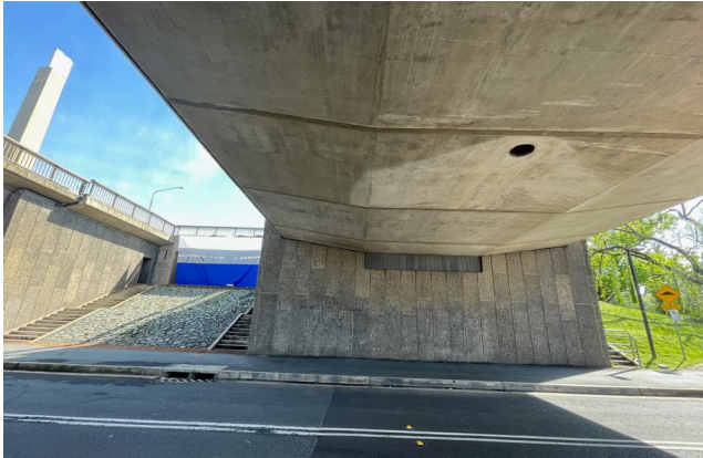
Figure 70: View of underside of eastern bridge on the city side.
