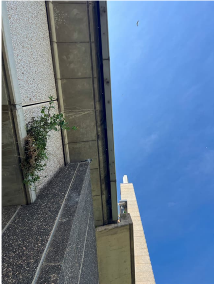
Figure 118: Detailed view of bridge connection and abutment.
