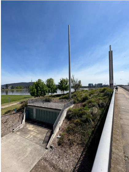
Figure 126: Substation on SW corner of bridge.
