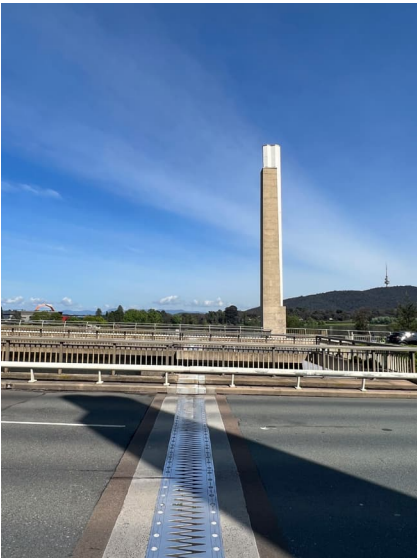
Figure 91: Movement joint of bridge looking west.
