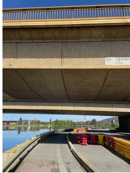
Figure 73: Detail shot of bridge edge showing precast panelling.
