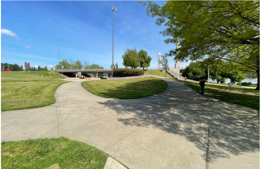
Figure 106: Rammed path access to bridge.
