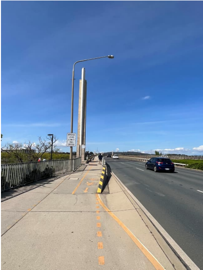
Figure 84: Approach to bridge southbound.
