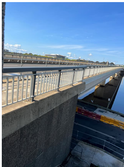
Figure 138: Edge detail abutment showing balustrade.
