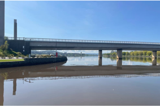
Figure 61: Commonwealth Avenue Bridge viewed from Henry Roland Park
