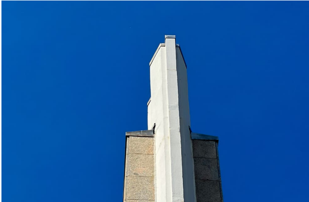
Figure 136: NW Pylon detail.
