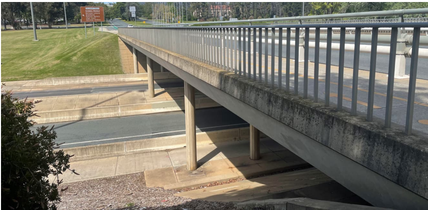
Figure 102: Flynn Drive Bridge detail.
