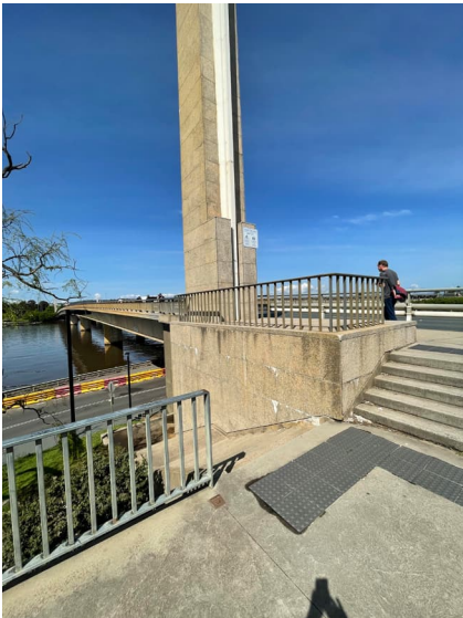
Figure 81: Stair arrangement around plinth to pylon.
