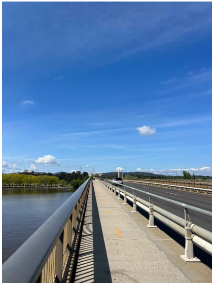
Figure 93: Pedestrian/ Cyclepath southbound.
