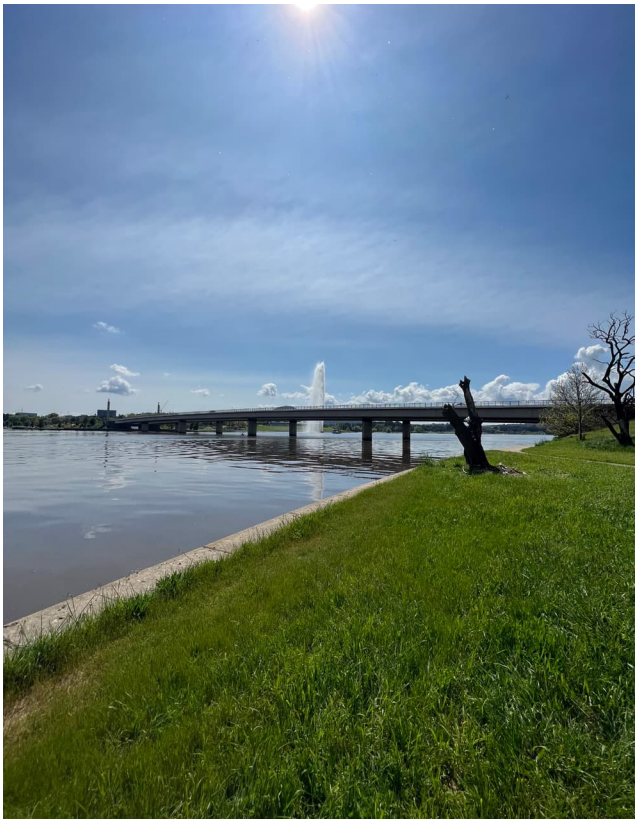
Figure 120: View of bridge from West Basin loop.
