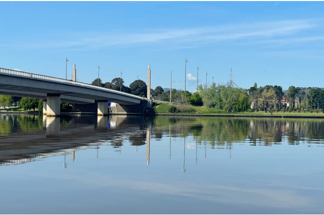
Figure 62: Commonwealth Avenue Bridge viewed from Henry Roland Park
