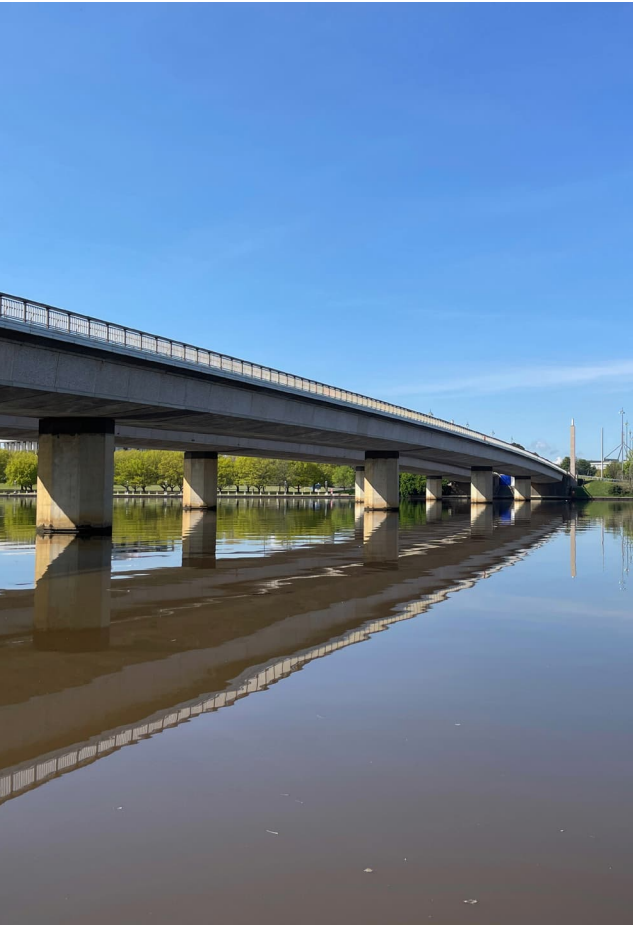
Figure 65: Commonwealth Avenue Bridge viewed from Barrine Drive looking towards Parliament.
