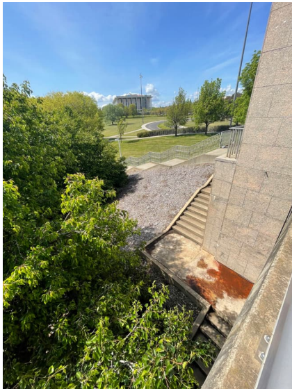
Figure 98: SE Pylon stair case.
