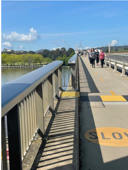
Figure 90: Balustrade junction on movement joint of bridge.
