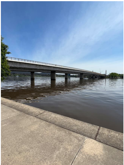
Figure 107: Bridge viewed from Australians of the Year walk.
