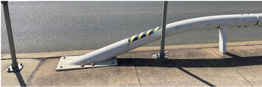
Figure 132: Termination detail of north bound barrier.
