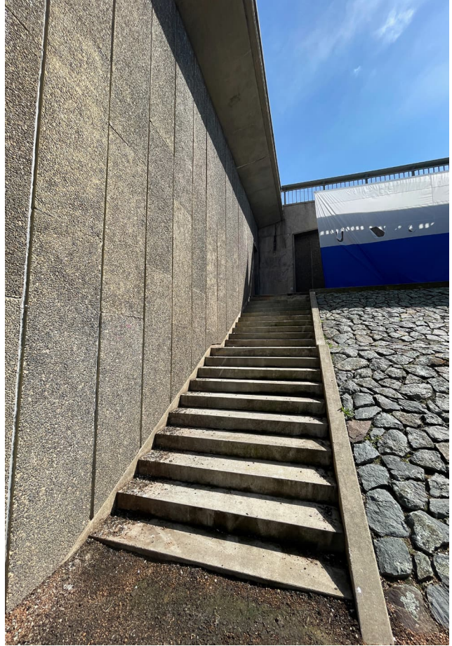
Figure 67: Stairs and embankment between the 2 bridges.
