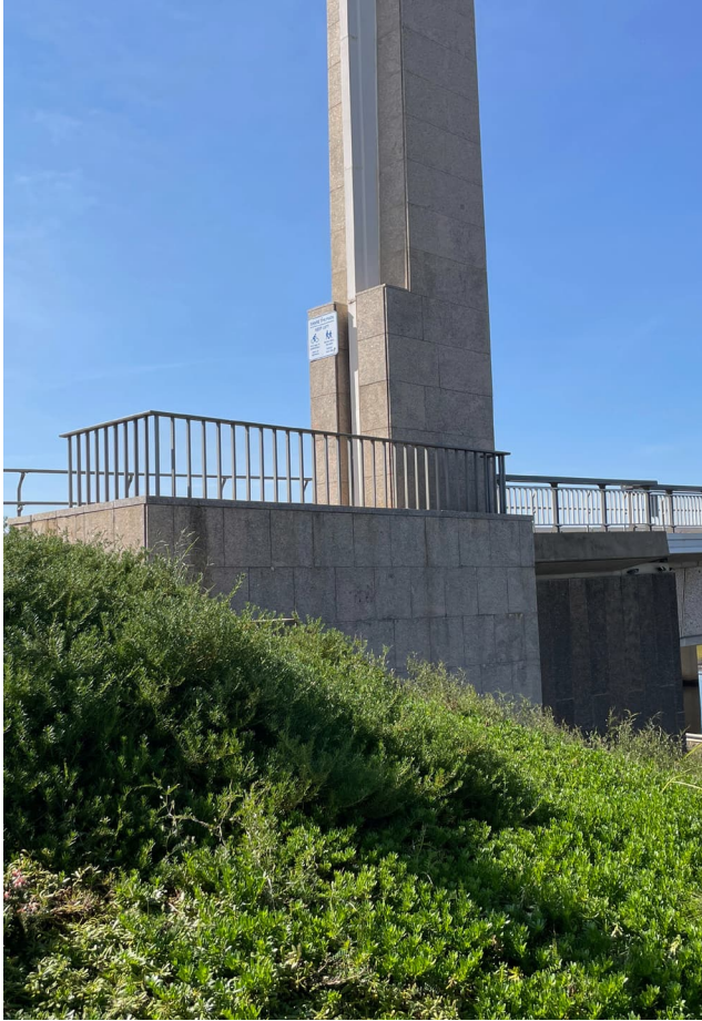
Figure 66: Base of Pylon situated NW of bridge.
