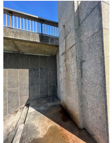
Figure 77: NE junction of bridge, stair and Pylon.
