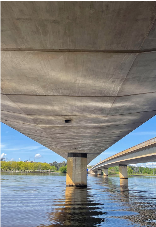
Figure 71: Centred view of eastern bridge soffit and pier.
