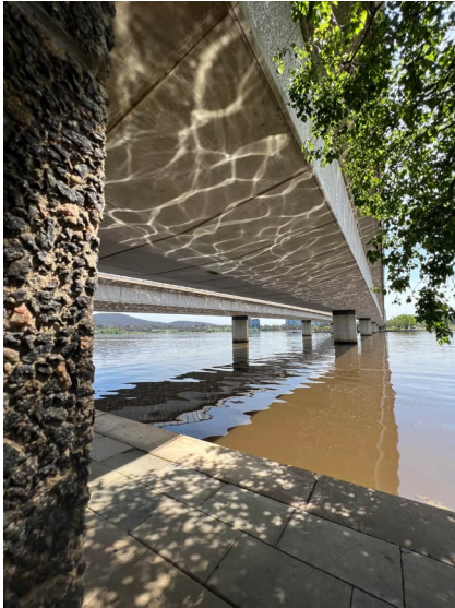
Figure 111: Detail bridge soffit with water reflection.
