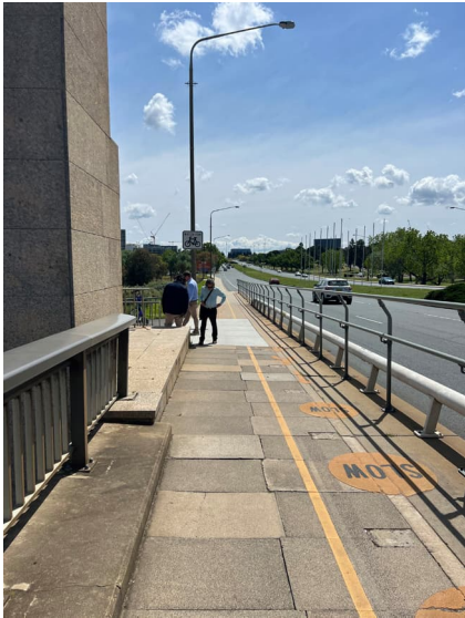
Figure 129: Pathway northbound on Civic side.
