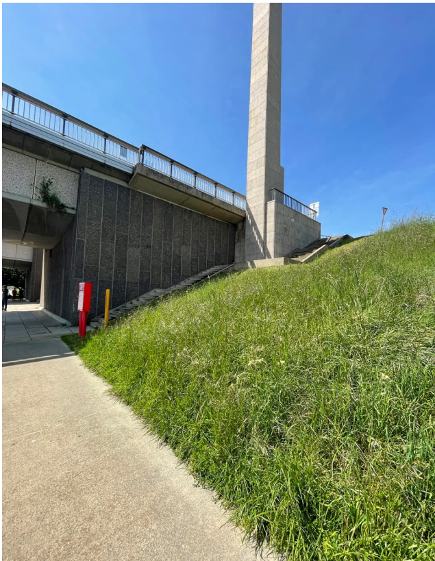
Figure 119: View of abutment.
