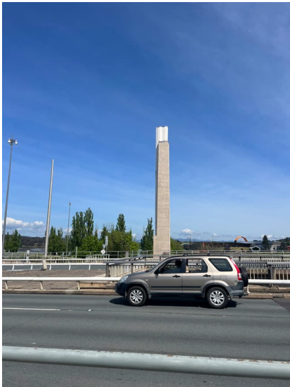
Figure 97: SW Pylon across lanes.
