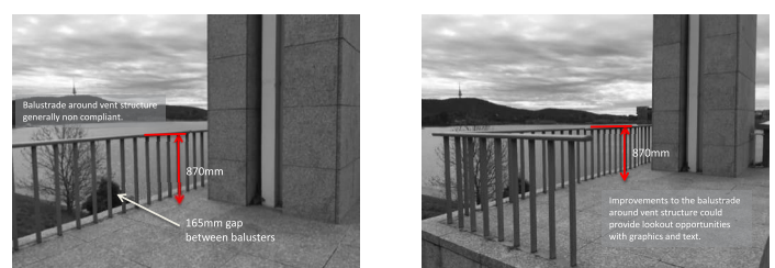
Figure 153: Existing balustrade around vent structure.
