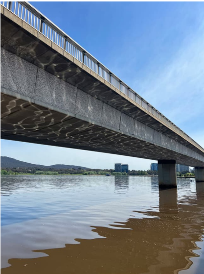
Figure 113: View of northbound bridge.
