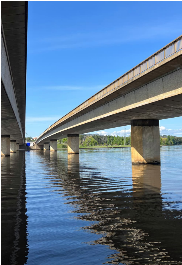
Figure 69: View of western bridge .
