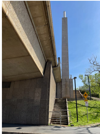
Figure 76: NE stair and Pylon.
