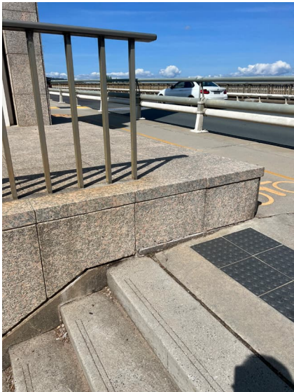
Figure 82: Top of Stair connection to Commonwealth Park.
