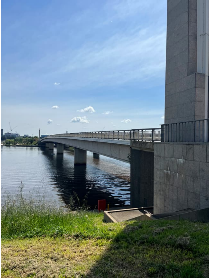
Figure 122: View northbound bridge.
