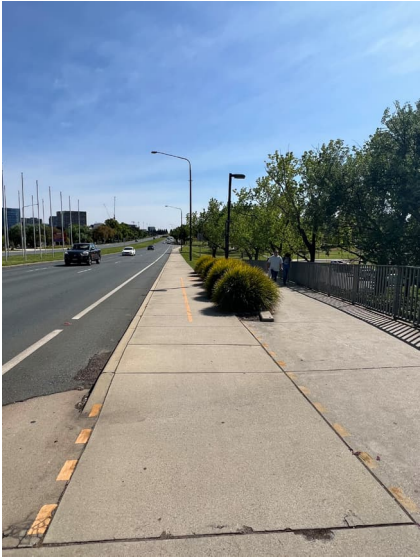
Figure 85: View of approach to bridge southbound.
