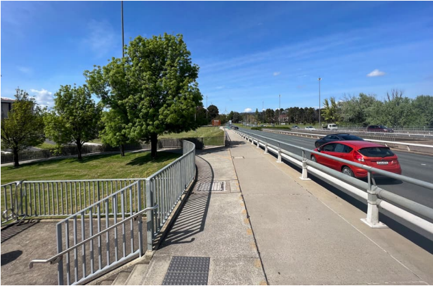
Figure 99: SE stair and ramp access to bridge.
