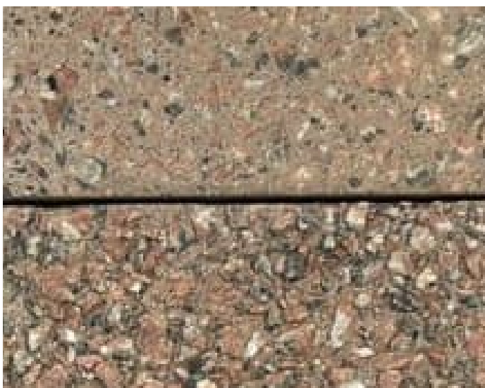
Figure 58: Precast cladding sample trials.
