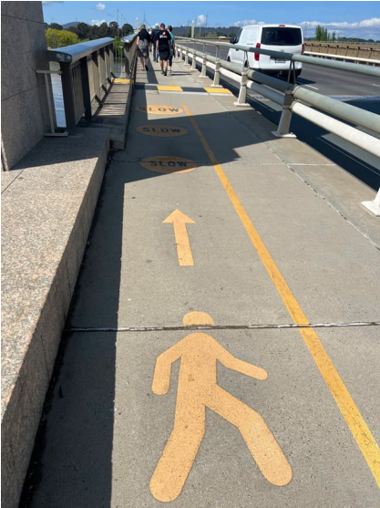
Figure 88: Pedestrian/ cycleway pinch point southbound.
