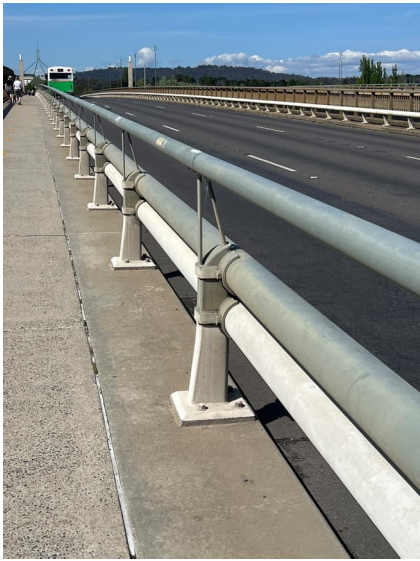
Figure 87: Barrier detail on southbound side.
