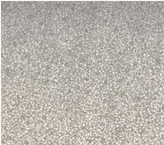
Figure 50: Existing washed concrete vertical cladding.
