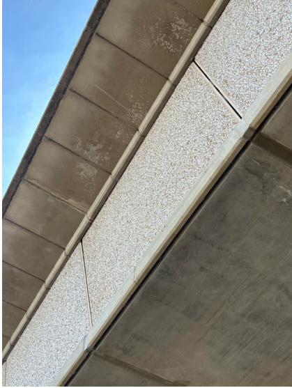
Figure 72: Detail shot of bridge edge showing precast panelling.
