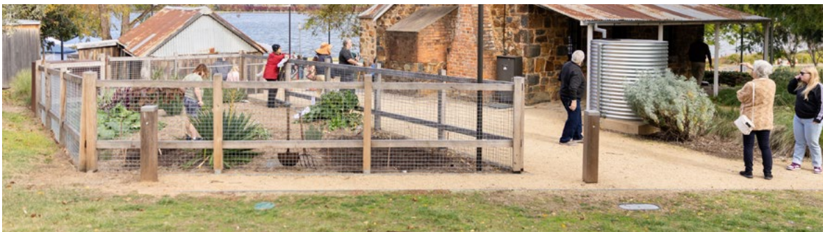
Blundells Cottage. Credit: National Capital Authority
