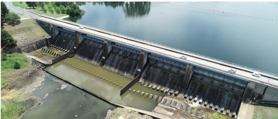
Scrivener Dam. Credit: National Capital Authority
