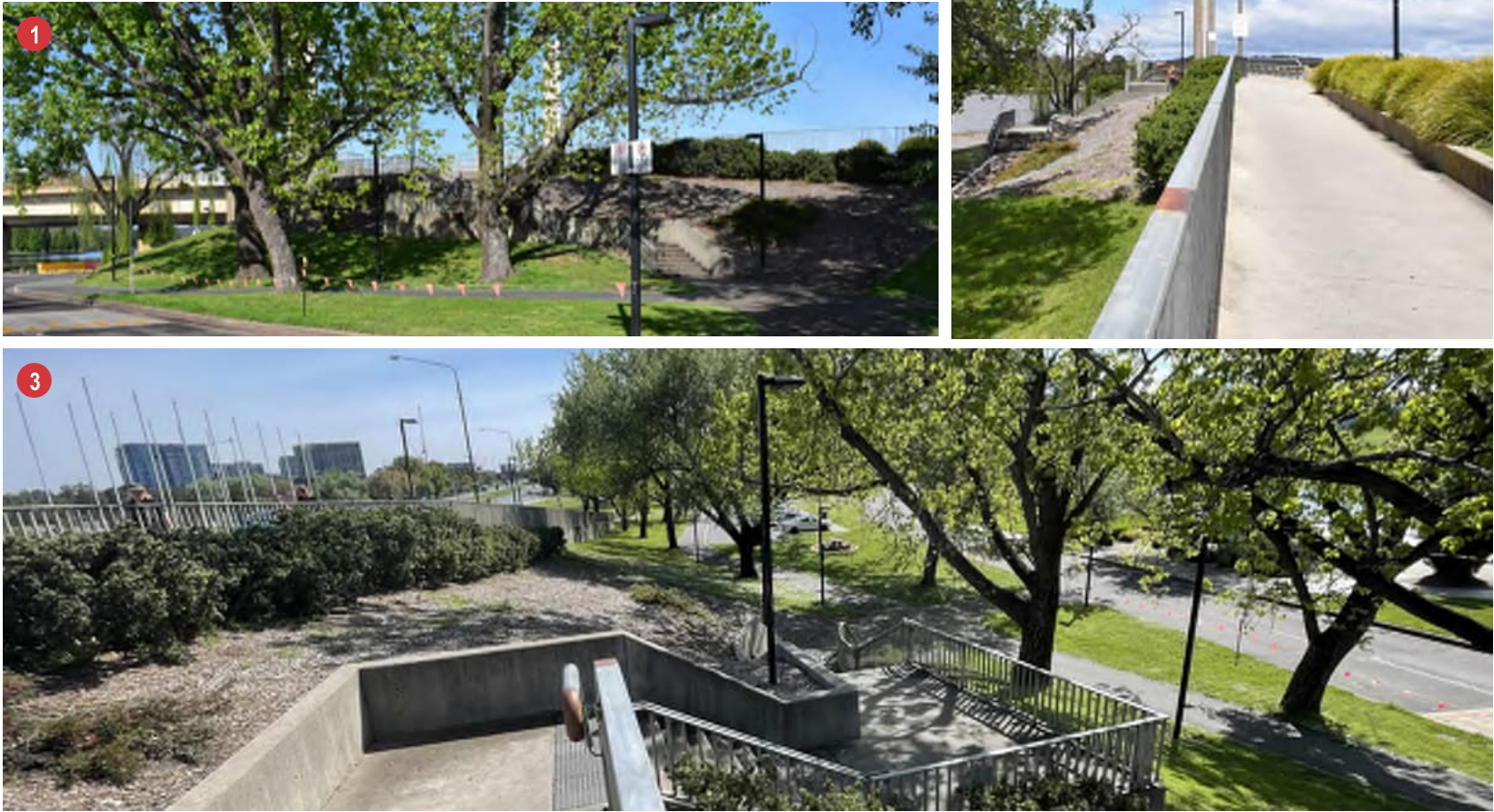
Figure 73: North-east approach existing site conditions
