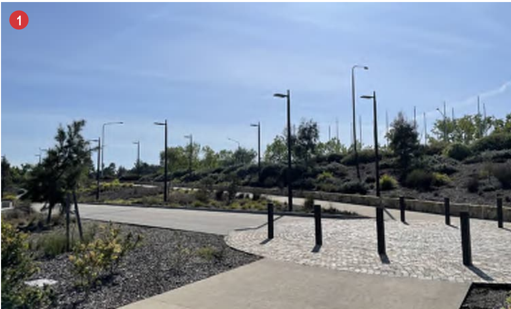
Figure 68: North-west approach existing site conditions
