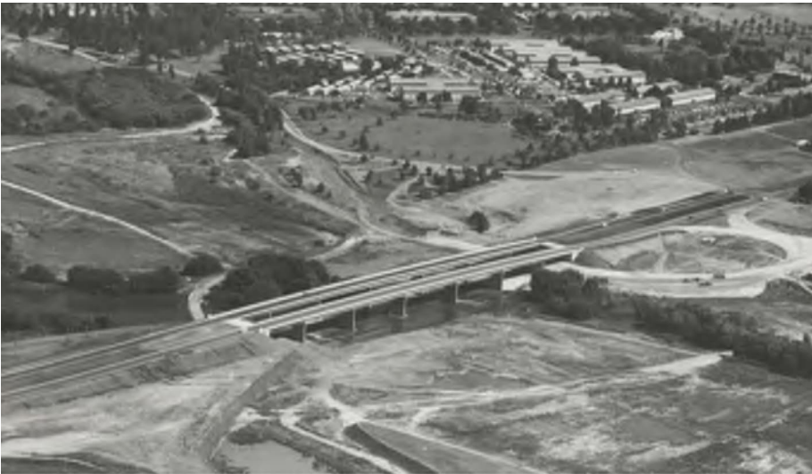
Figure 1: The Bridge was constructed in early 1960s
