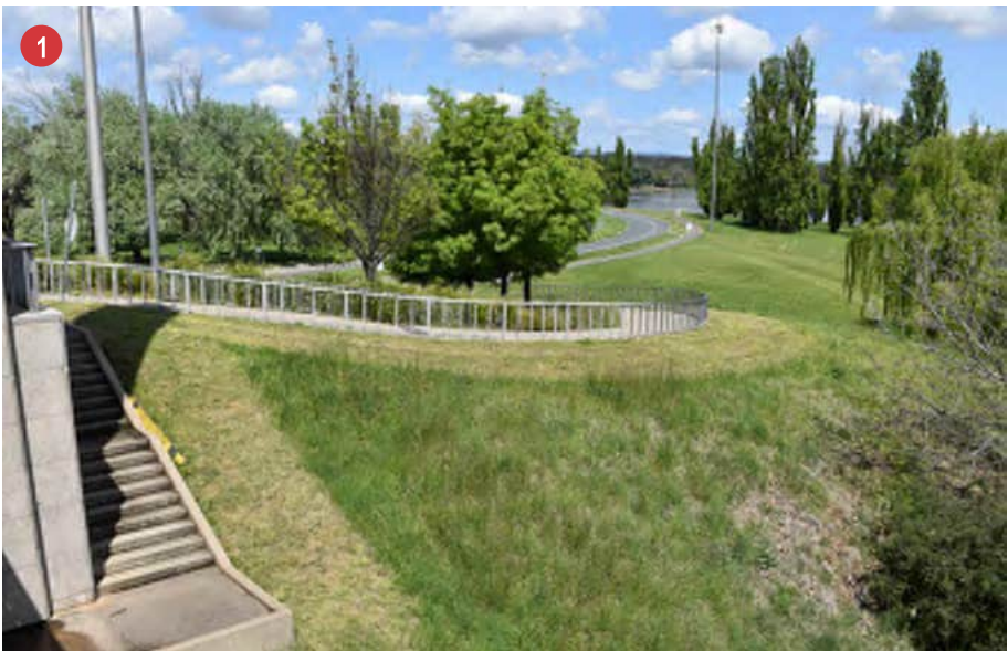
Figure 80: South-west approach existing site conditions
