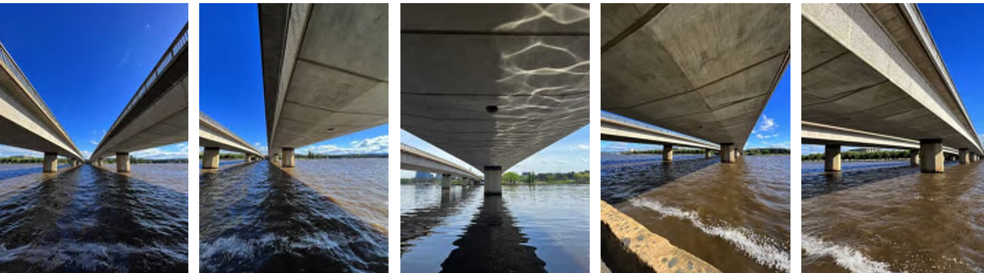
Figure 46: Different viewpoints under the northbound Bridge looking south
