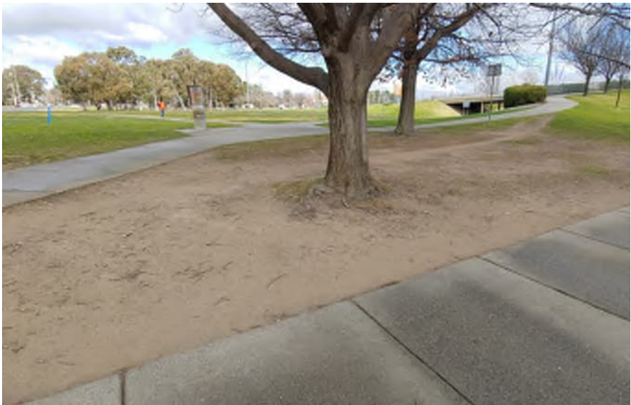
Areas that enable cut-throughs between formal paths result in desire lines and turf die-back
