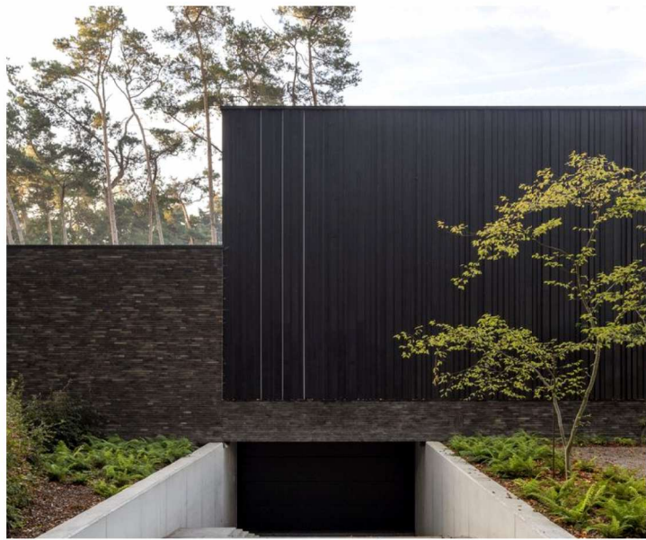
M.01 CHARCOAL VERTICAL TIMBER CLADDING
