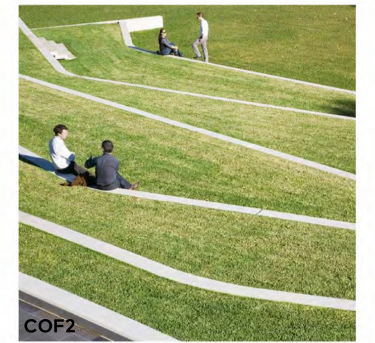
CONCRETE STEPS AND RETAINING CLASS 2 OFF-FORM CONCRETE
