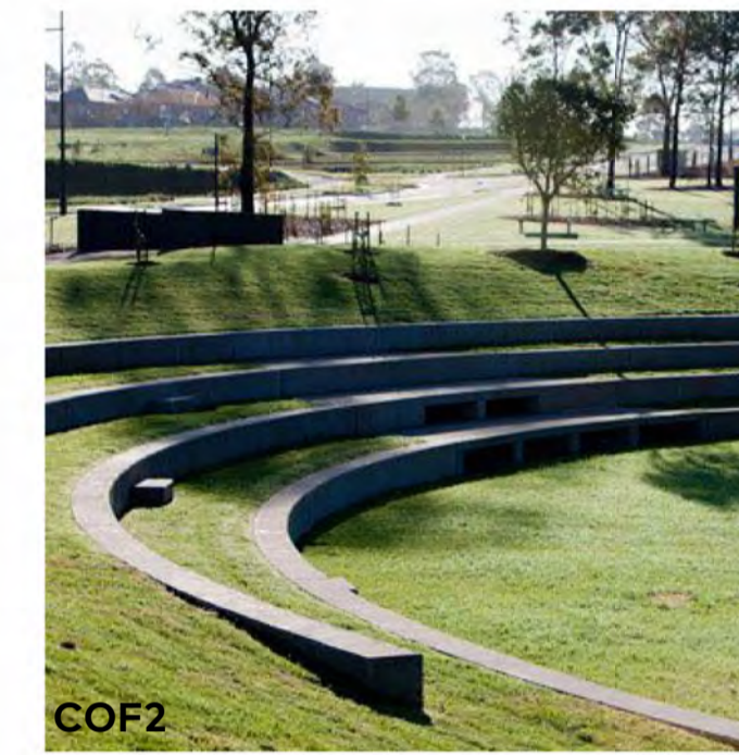
CONCRETE STEPS AND RETAINING CLASS 2 OFF-FORM CONCRETE
