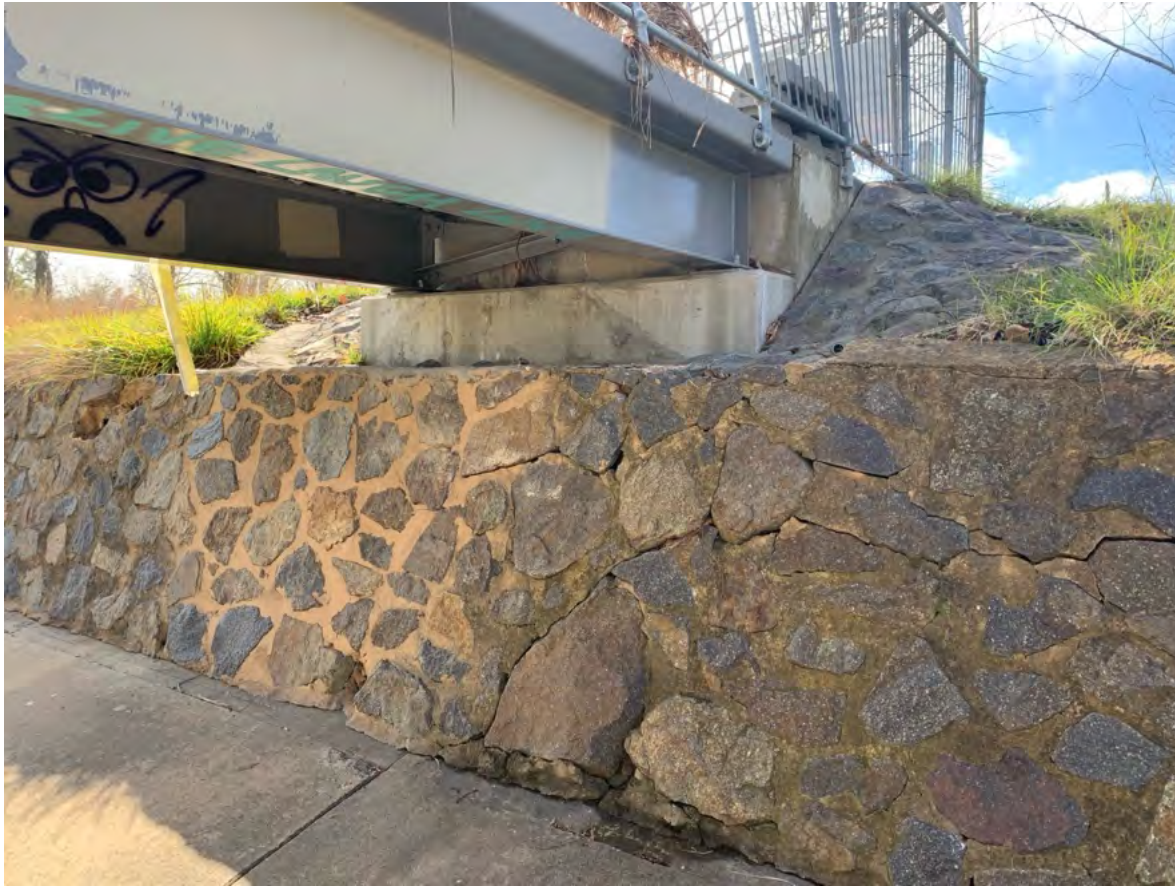
Figure 7 - Foundation & I-beams active travel bridge directly upstream of the proposed development
