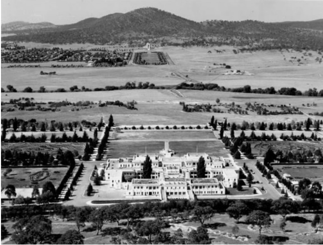
Figure 53. Vista looking North in c1939 from above Capital Hill
