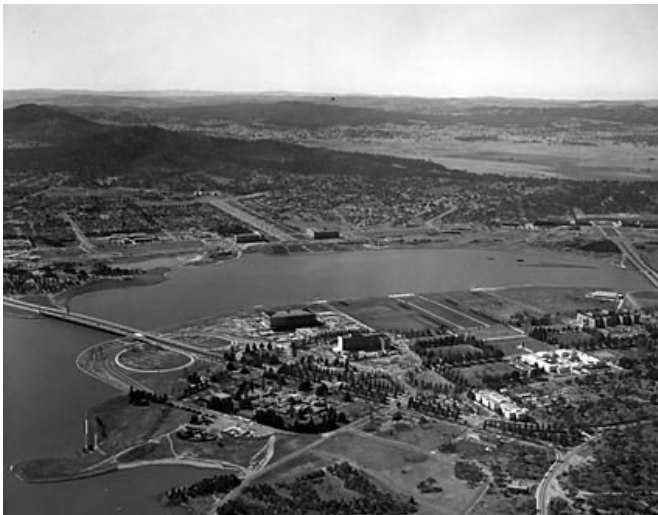
Figure 75. Vista looking Northeast in 1967
