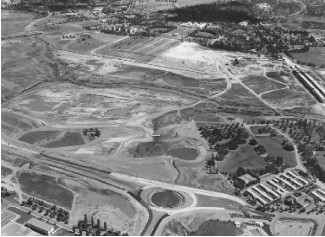
Figure 63. View South over Molonglo floodplain during construction works for lake, 1963
