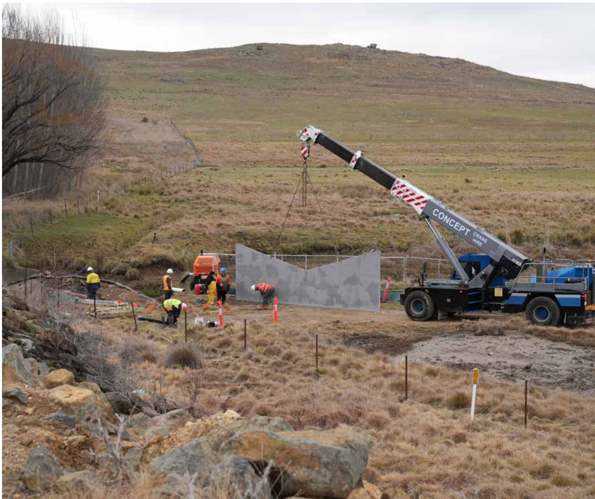
Jerrabomberra Weir Project
