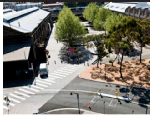
AUSTRALIAN TECHNOLOGY PARK, SYDNEY DEMONSTRATES COORDINATION OF SERVICE INFRASTRUCTURE
