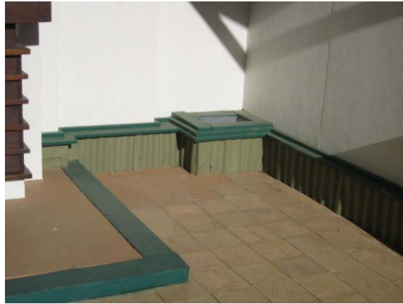
Figure 32: Wall detail showing corrugated-iron edging and planter box. (Source: GML, 2011)
