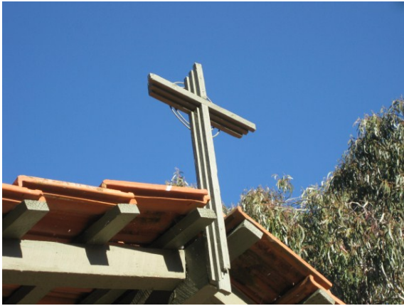
Figure 31: Timber cross on ridge of the roof. (Source: GML, 2011)
