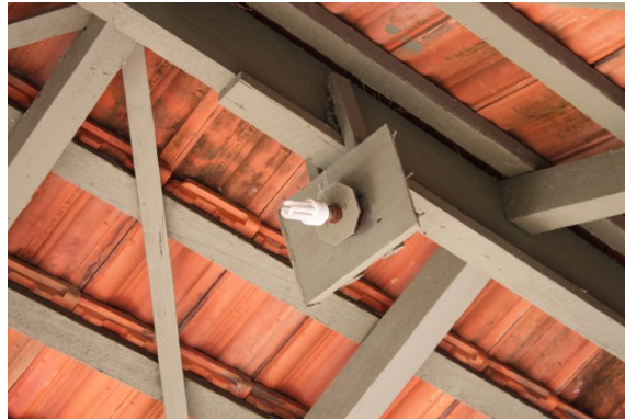
Figure 36: Light bulb inside the Chapel. (Source: GML, 2011)
