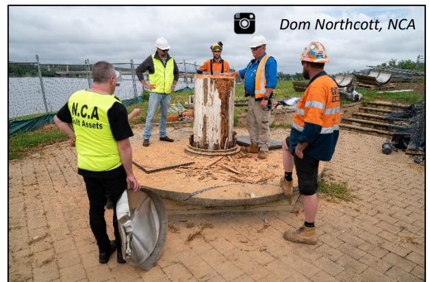
NCA staff and the Flagpole project team with the flagpole base after it was fell by an arborist
