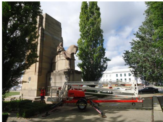
Figure 5.10 View of the memorial, located between two Lombardy poplars. (Source: GML 2013)
