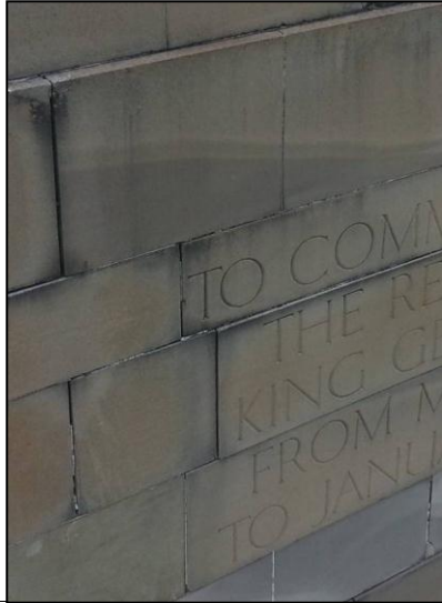
Figure 5.3 Typical weathering of mortar joints.
