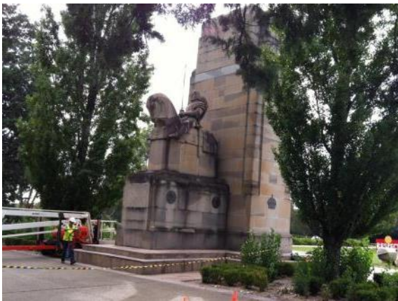
Figure 2.8 View from the southwest toward the memorial showing Saint George upon his horse. (Source: GML 2013)
