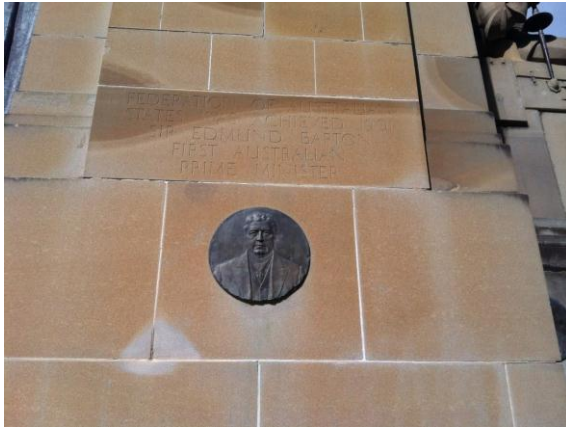
Figure 2.12 Bronze plaque of Sir Edmund Barton on the North Elevation. (Source: GML 2013)
