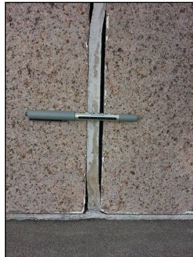
Figure 5.2 Detail of granite steps, showing widening of the centre joint.
