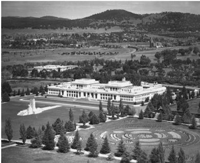
Figure 5.12 1948 view of Old Parliament House and King George V Memorial (without surrounding trees and monumental in the space), which shows the early linear planting of Lombardy poplars and other exotics adjacent to the circular formation of the National Rose Garden. (Source: National Archives of Australia, A1200, L11331A)
