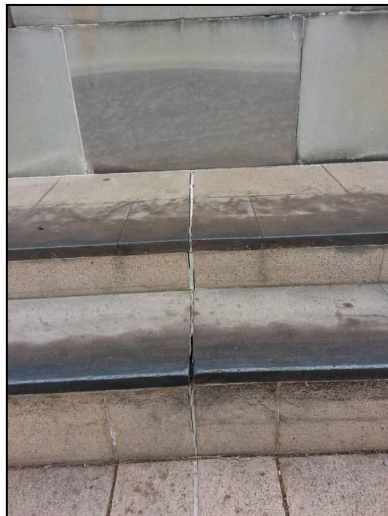
Figure 5.1 Granite steps showing the widening centre joint (and staining from skateboarders wax).
