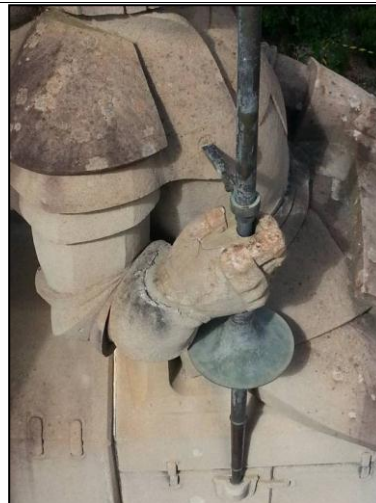
Figure 5.6 Cracking at the wrist of the Saint George stone sculpture.
