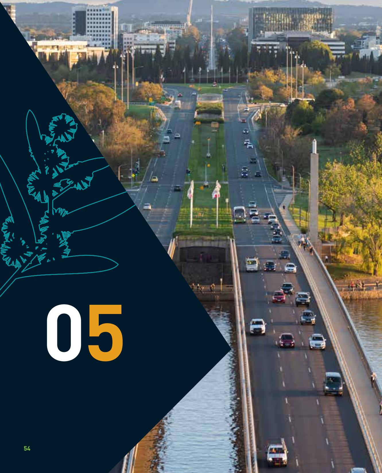
Commonwealth Avenue Bridge, Parkes, photographed by Martin Ollman
