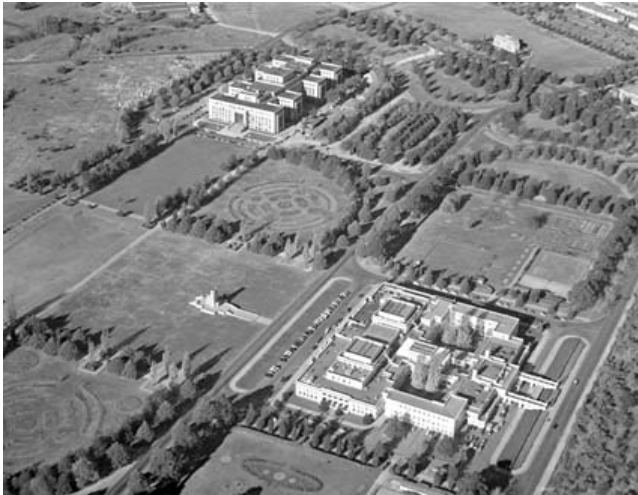
Figure 51. Aerial view of Parkes Place, 1957
