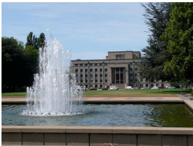
Figure 36. The John Gorton Building viewed from within the cross-axis in Parkes Place
