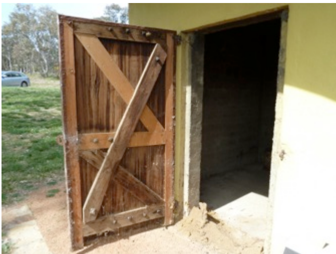
Figure 9. Hut doorway open with evidence of termite activity at base
