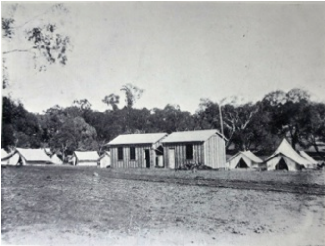
Figure 20. The timber and malthoid huts with the water tank between them circa May 1910, before the Plan Room (Surveyors Hut) had been added
