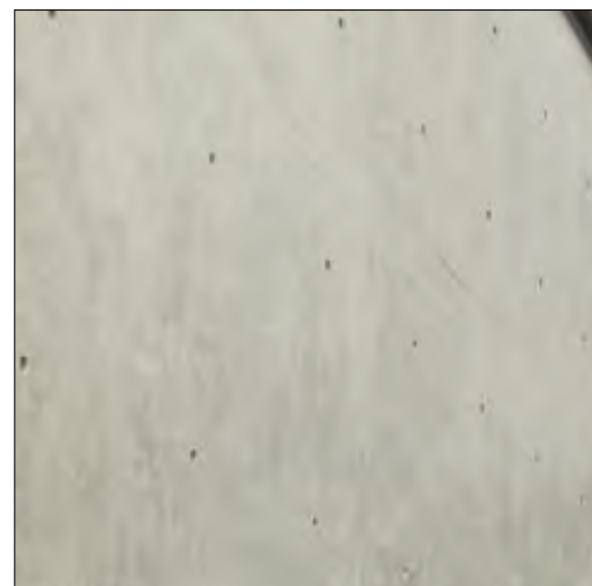
In situ concrete with high quality natural finish Code: CONC1 Colonnade columns Colour: Natural Light Grey finish
