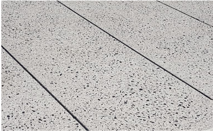
Figure 3: Quarried basalt stone exposed aggregate and saw cuts give a contrast to the 2700mm wide margin
