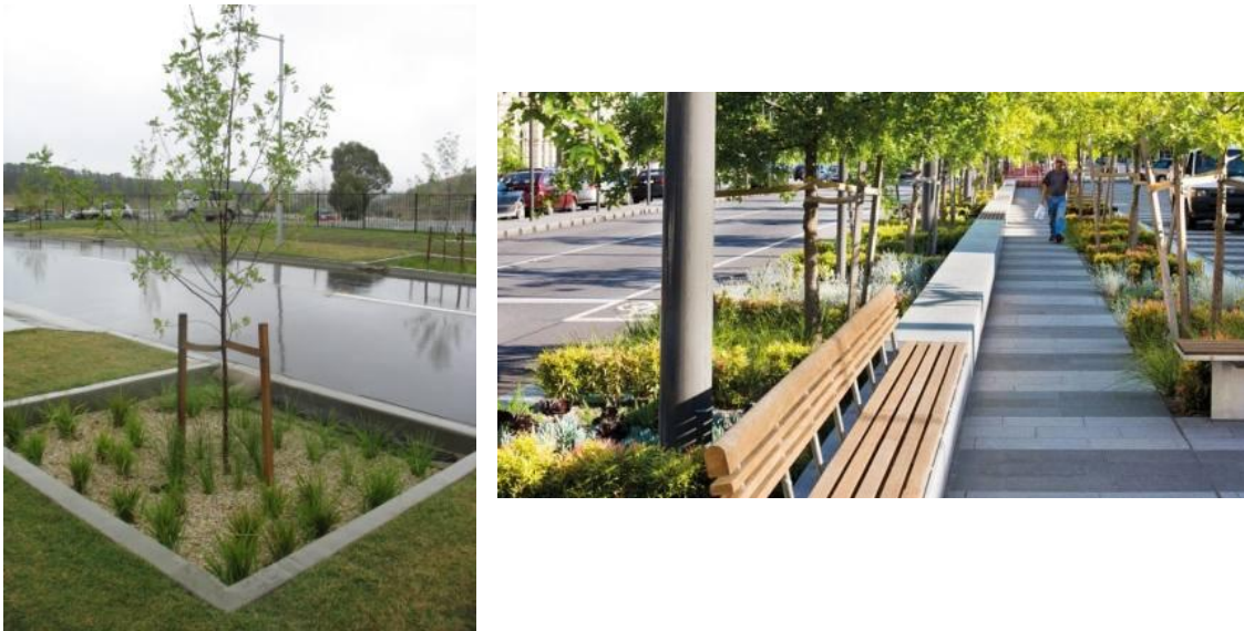
Figure 11 Bioretention Tree pit at Crace, ACT (left) and Bioretention containing Street trees in Central Dandenong (Lonsdale Street) (right)
