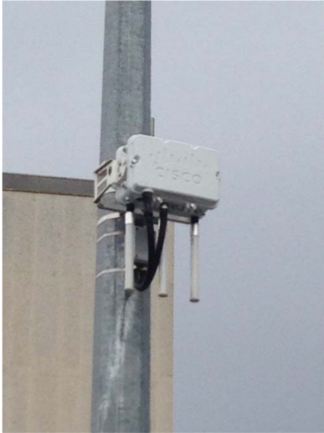
Figure 6 – Cisco Wi-Fi unit attached to existing lighting pole in the Magistrates Court Car Park
