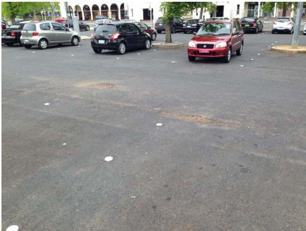
Figure 5 – Example of pavement damage in the Magistrates Court Car Park
