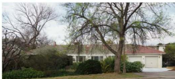
Existing dwelling at 10 Canterbury to be demolished
