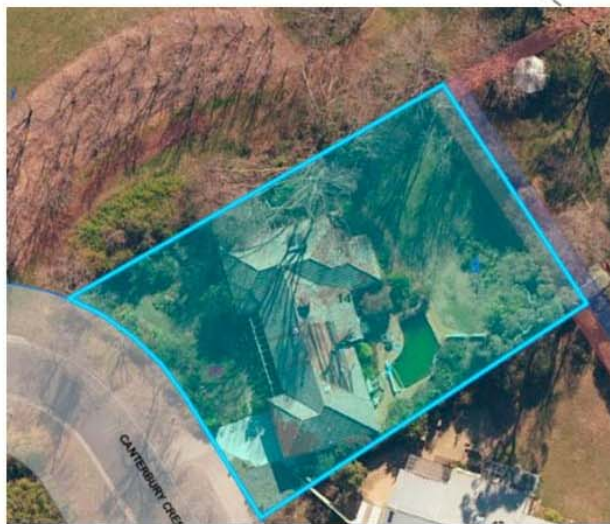
Existing dwelling at 10 Canterbury to be demolished
