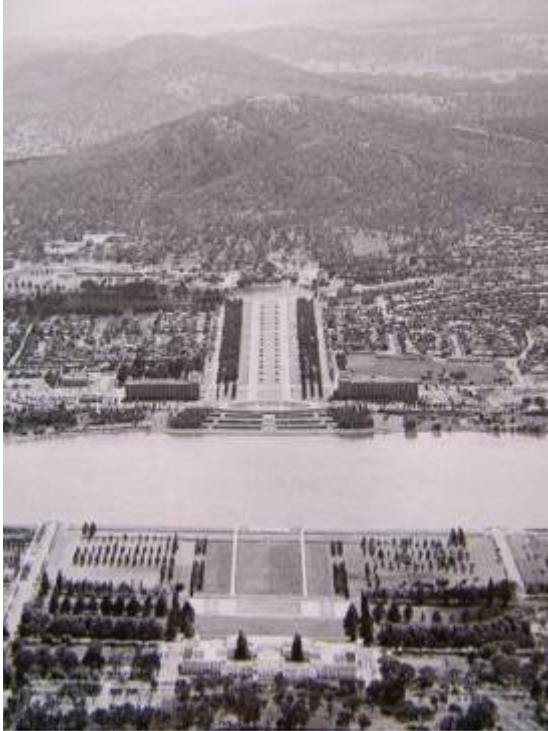
Figure 79. Detail view along the Land Axis with completed Anzac Parade treatment
