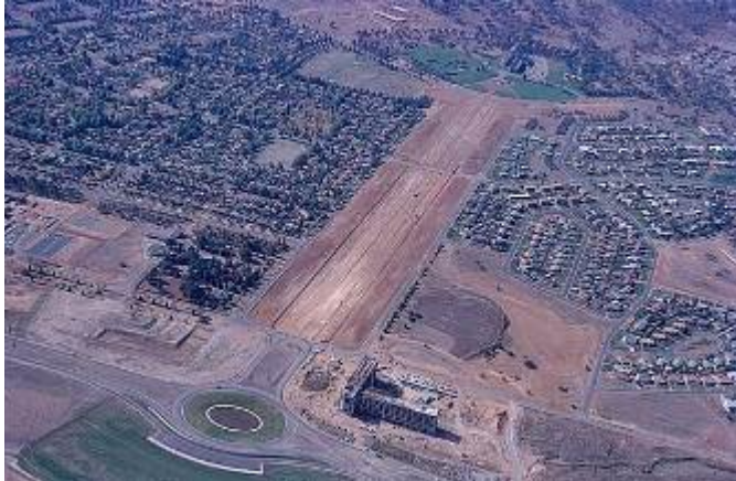
Figure 37. Aerial view of Anzac Parade looking North, under construction, c1965
