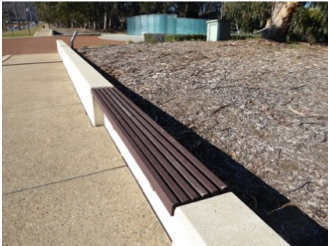
Figure 9. Typical concrete wall and timber seat on Anzac Parade with the Australian Service Nurses National Memorial in the background Source: Duncan Marshall
