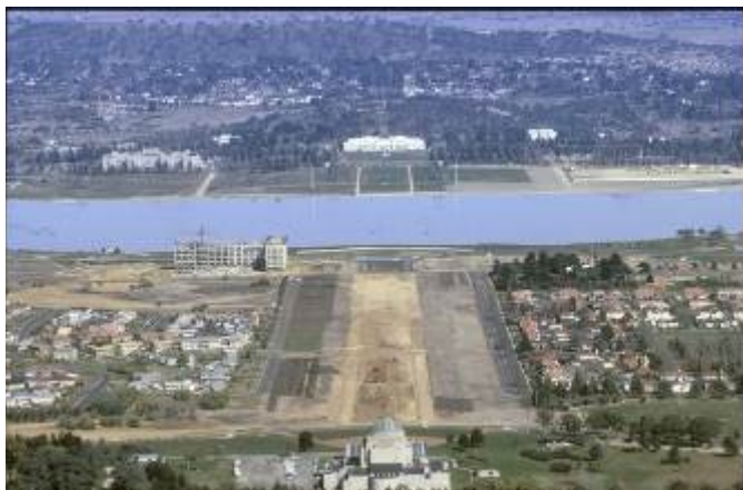
Figure 89. Earthworks showing both carriageways of Anzac Parade, Canberra, photo by Richard Clough, c1962
