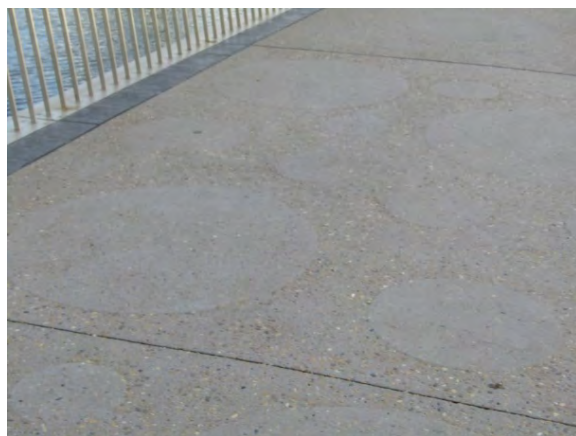
Figure 3.13 Detail of the surface of the bridge, which is exposed aggregate concrete with circles incorporated into the finish. (Source: GML, July–August 2019)
