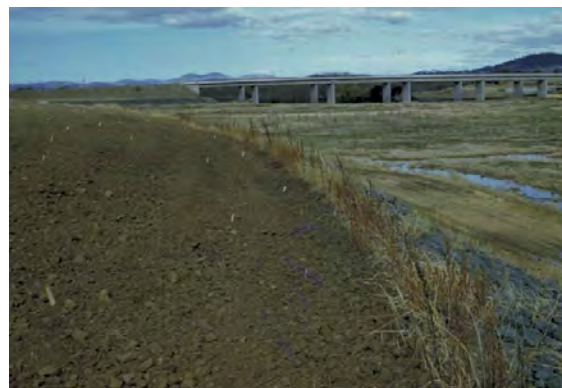
Figure 2.8 Detail of the Aspen Island constructed platform showing rock foundation and topsoil, c1960–1962. (Source: National Library of Australia, PIC P2214/211)
