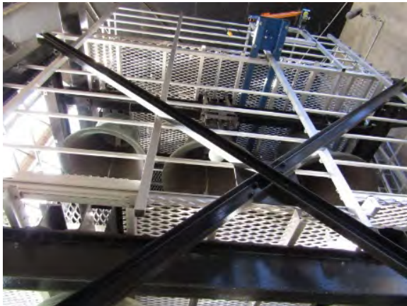
Figure 3.32 View of the Bell Chamber showing the steel frame and mesh gangway system. (Source: GML, July–August 2019)
