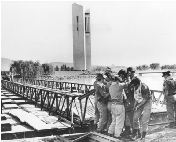
Figure 2.21 Army engineers from Holsworthy, NSW, dismantling floating bridge, c1970. (Source: ACT Heritage Library, Ref. 005398)
