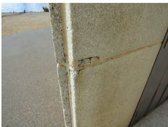
Figure 3.24 Detail of cracking and discolouration on inner façade of shaft. (Source: GML, July–August 2019)
