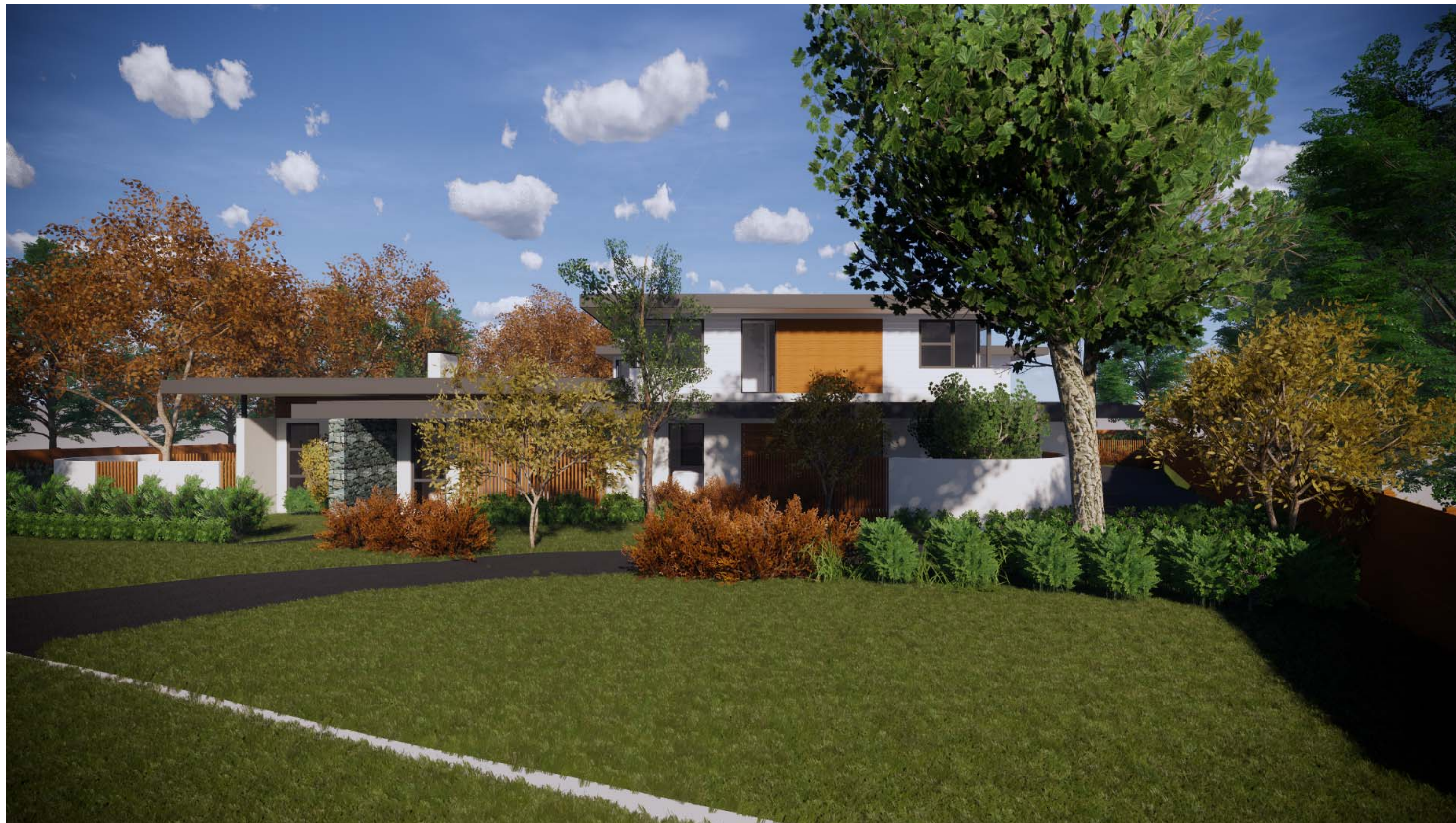
STREET VIEW TO UNIT 3
