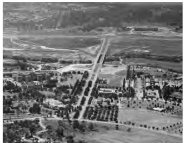
▲ Kings Avenue nearing completion, early 1960s
