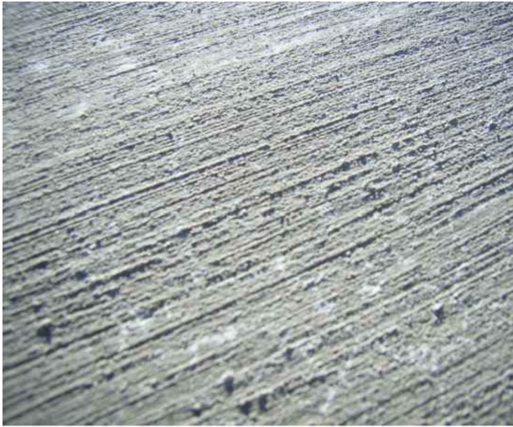
CON2 Concrete broom finish
