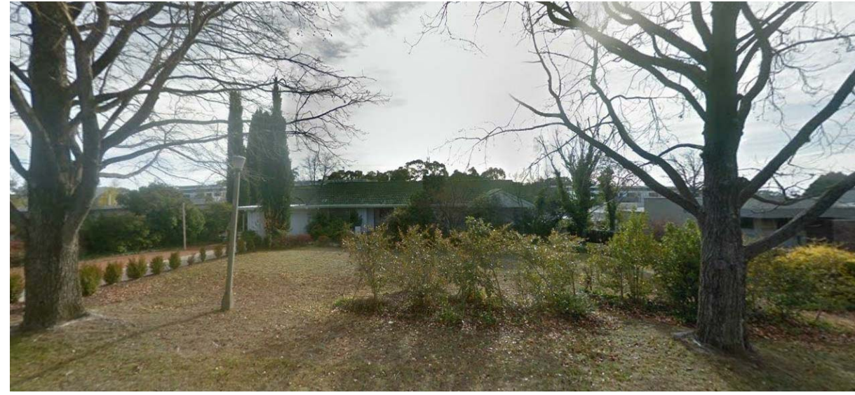
NO.12 SOMERS CRESCENT
