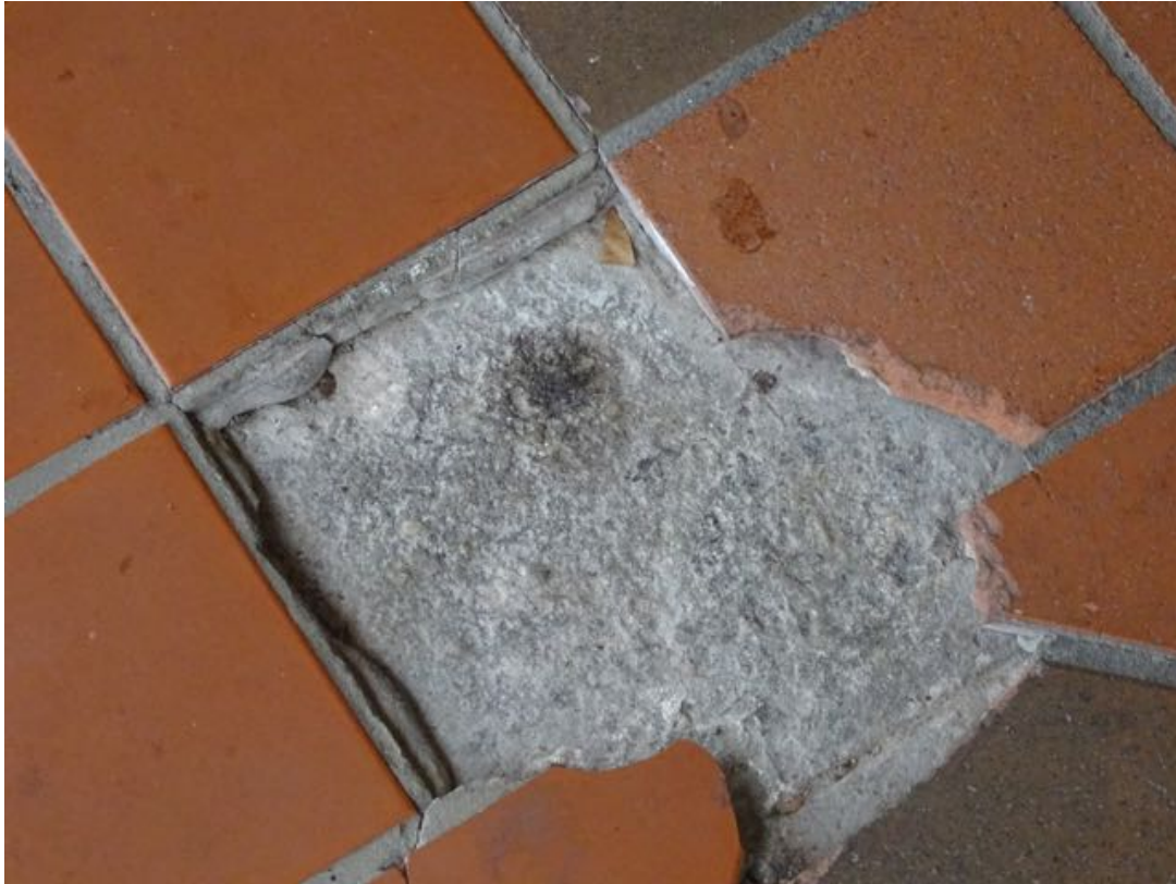
Photo 14: Original paving visible under quarry tiles, Alinga St Source: PLA 2017: Note thicker cementitious tile bed in this instance
