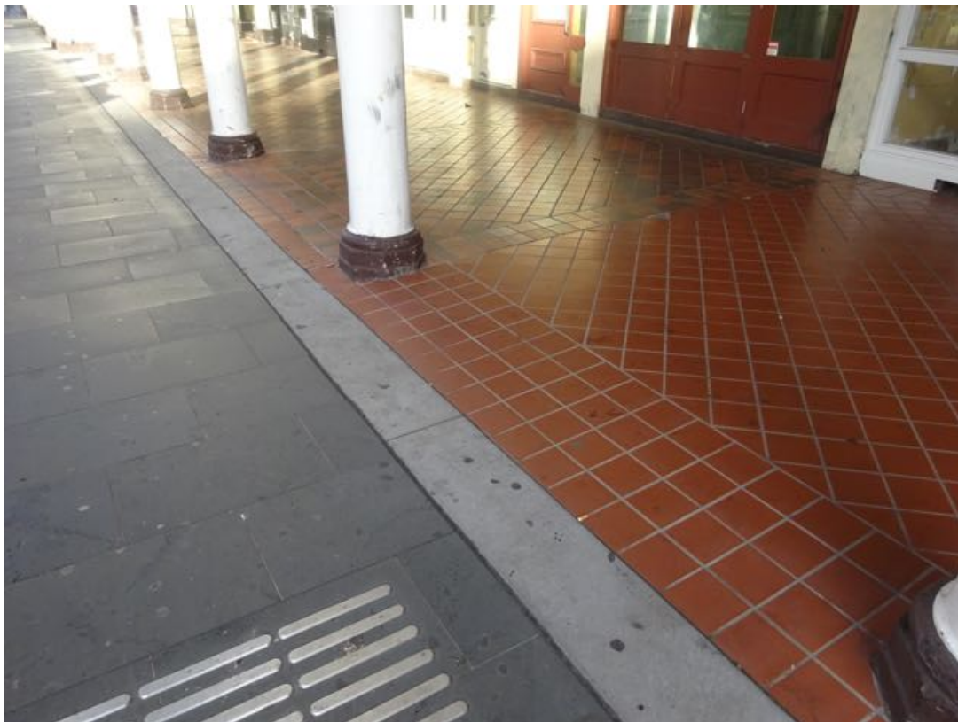
Photo: Raised verge Alinga St Source: PLA 2017-07-05: Note flush broomed concrete strip at former perimeter step location
