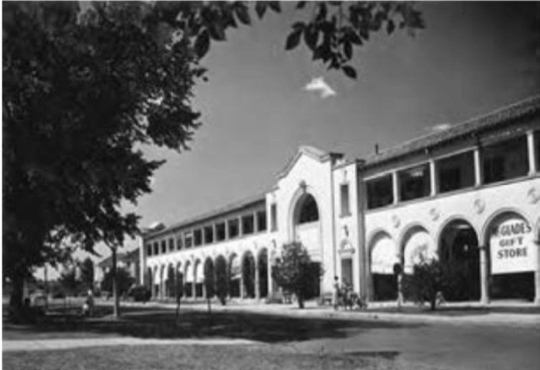
Photo 4: Sydney Building from Northbourne Ave median 1951 Source: ACT Heritage Library, Dept of Capital Territory Collection, 009165 Note verge treatments
