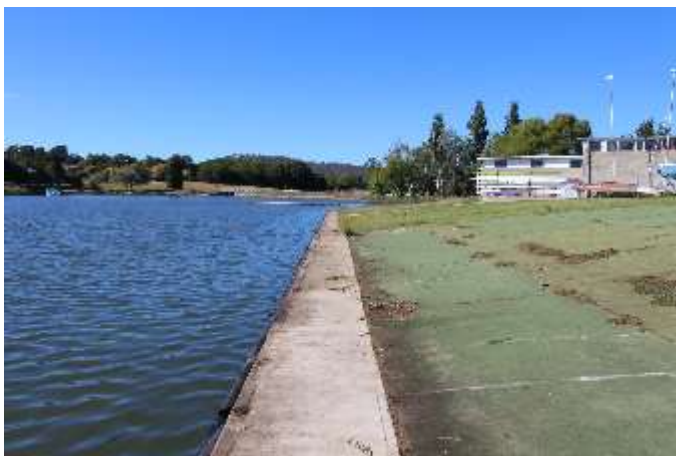
View from lakeside in front of existing shed looking South across Yarralumla Bay from Girl's Grammar rowing club location (Fig 16)
