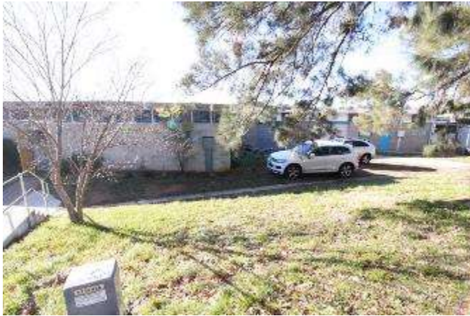
View of front of CRC shed from Alexandrina Drive (Fig 11)
