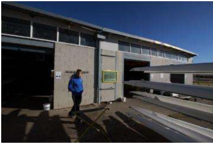
Boat handling area outside front of current CRC shed (Fig 15)
