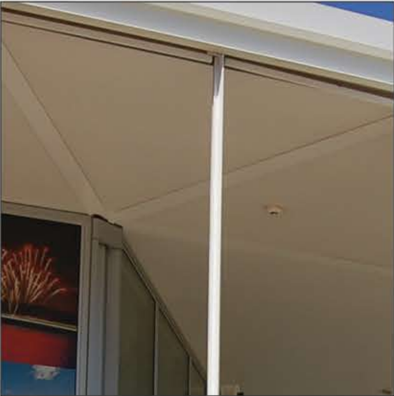
SOFFITS: PAINTED 6mm THICK FC SQUARE EDGED CAULKED JOINTS.
