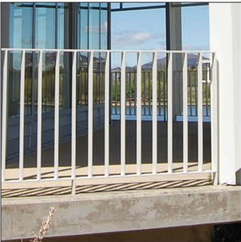
DECK BALUSTRADES: BALUSTERS 50X10 MS. FLATS @ 120 CTS. HANDRAIL 75X16 MS FLAT. ALL FULLY WELDED. BALUSTERS WELDED TO DECKING EDGE 380 PFC. PAINT FINISH 'WHITE' TO MATCH EXISTING STEEL WORK.
