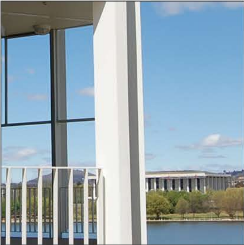
AWNING ROOF TO MAIN DINING SPACE: FOLDED & FABRICATED IN FULL WIDTH SECTIONS FROM 4MM THICK MILD STEEL PLATE. INTERNAL FACES PRIMED WITH INORGANIC ZINC PRIMER AND EXPOSED SURFACES PAINTED WITH 2 PACK SYSTEM HIGH DURABILITY EQUAL TO AMERON PAINTS (PPG INDUSTRIES).
