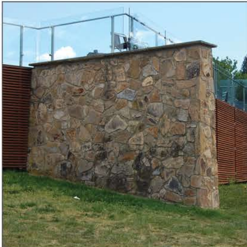
STONE WALLS: PIALLIGO STONE RANDOM RUBBLE TO MATCH EXISTING. DEMOLISHED STONE FROM EXISTING DECK BASE WALLS TO BE RE-USED.
