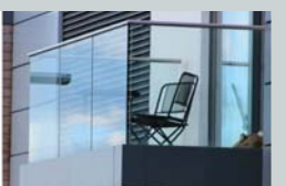
GL-1 - Clear glass and metal handrail: Frameless handrail with compression plate fixing to slab edge and SS U-channel top
