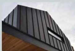
WT-2 - Black metal cladding: standing seam cladding
