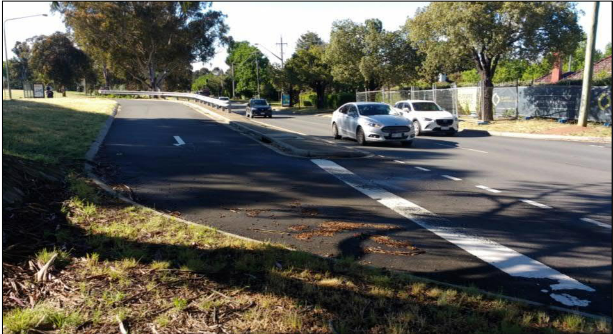
Figure 4: Limestone Avenue (right turn lane/ramp)
