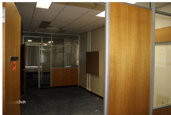
Figure 2.52 Sample internal office in Building 1, showing timber partition walls and highlight glazing panels.
