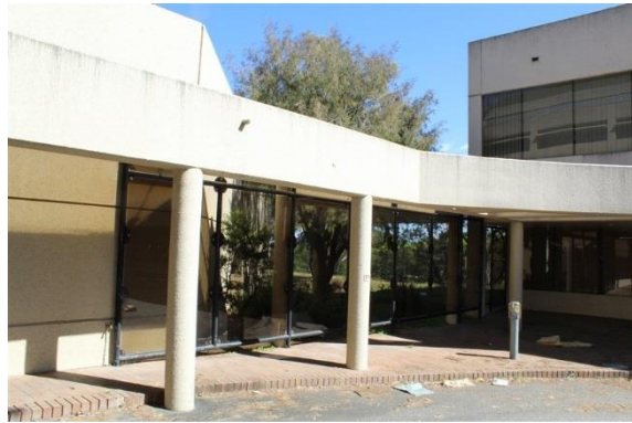
Figure 2.48 Concrete framing structure visually linking the three buildings. Note also later added glazed panels.
