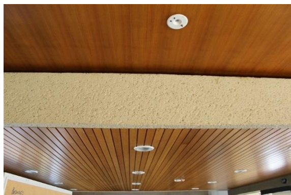
Figure 2.50 Lowered timber panel ceiling in the single storey lobby building (joining Buildings 1 and 2).
