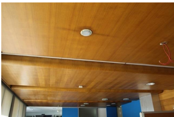
Figure 2.49 Moulded timber plywood ceiling in the single storey lobby building (joining Buildings 1 and 2).
