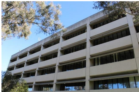
Figure 2.36 South facade of Building 1 showing concrete 'sunshade' awning detail.
