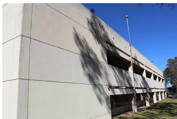
Figure 2.44 North facade of the two-storey office Building 3, showing concrete detailing and sun shades.
