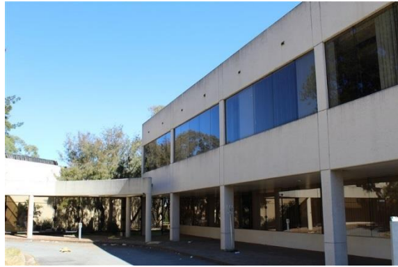
Figure 2.46 South façade of Building 3, showing concrete framing structure visually 'joining' it to Building 2.
