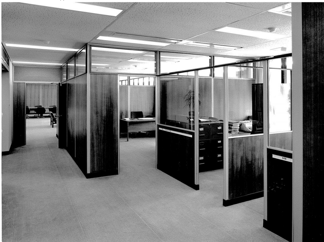
Figure 2.17 Interior fitout of the CSIRO Headquarters (Building 1), showing timber partition office walls with highlight glazing, and original furnishings. (Source: Mark Willett, MSJ Group)
