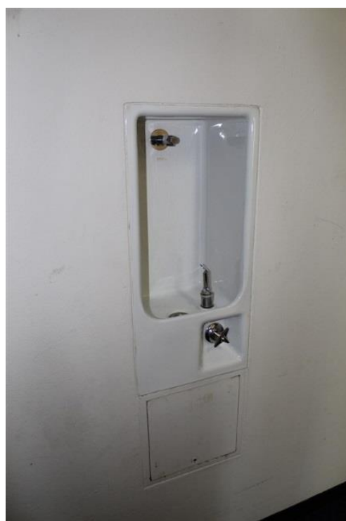
Figure 2.56 Built-in drinking fountain in the wall adjacent the kitchenette (evident on multiple floors).
