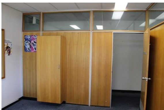
Figure 2.53 Sample office in Building 1, showing timber partition walls, highlight glazing panels, and custom built coat cupboard.
