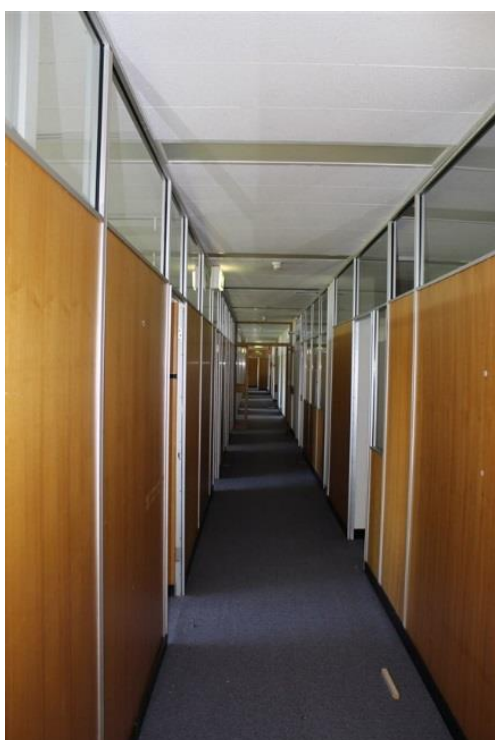
Figure 2.55 Corridor in Building 1, showing offices positioned either side with timber partition walls and highlight glazing panels.
