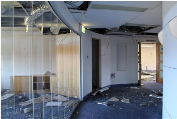
Figure 2.59 Later addition (circa 2000s) glazed and curved wall fitout at western end of floor five within Building 1.
