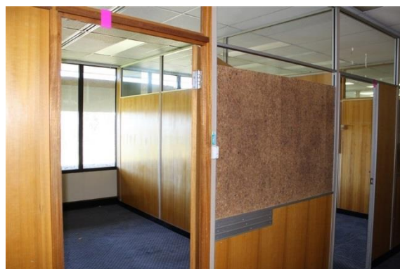
Figure 2.54 Sample office in Building 1, showing timber partition walls and highlight glazing panels.
