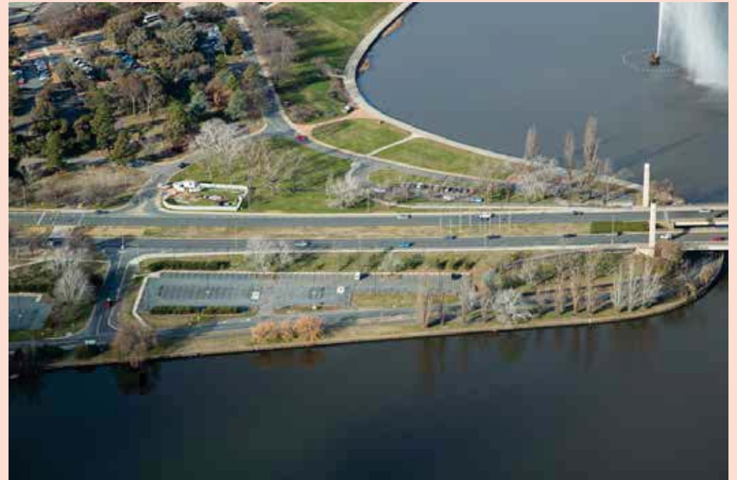
Surface carparks dominate West Basin
